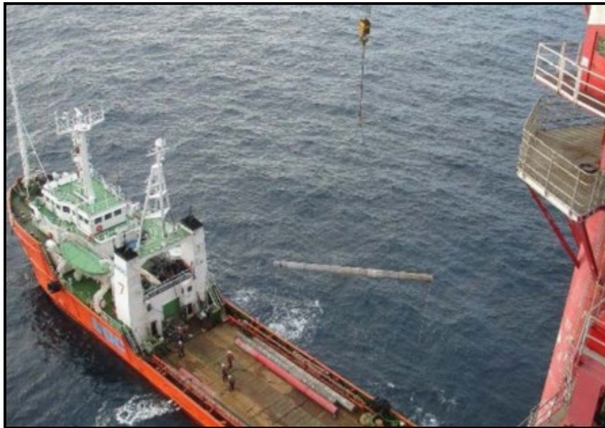
Figure 2.2-2. Example Cut Conductor Pipe Being Offloaded to Transport Vessel
