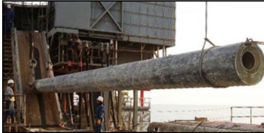
Figure 2.2-1. Example Cut Conductor Pipe Being Placed on Platform Deck
