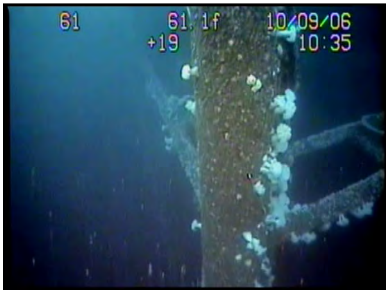
Figure S.16-2. Video Still of Epibiota on Northwest Jacket Leg (Depth Approximately 200 ft [61 m])
