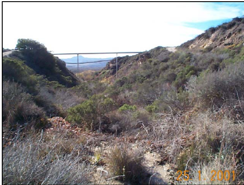
Figure 3.4-2 Photograph of Pipeline (foreground) Route Crossing Small Drainage Feature Near Basin 4
