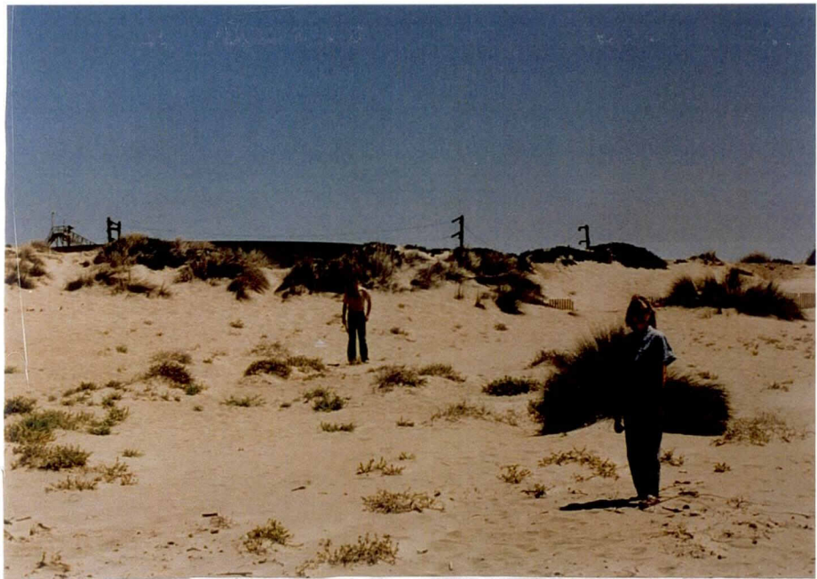
Plate 16. Site of seaward end of conduit under the dunes (Chris Culver in background) and onshore tie-in point (MBC biologist in foreground).
