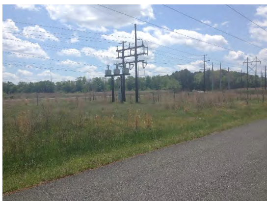
LOOKING SOUTHWEST FROM GATE A ROAD IN SOUTHWESTERN PORTION OF STUDY AREA. OLD FIELD AREAS AT LEFT.
