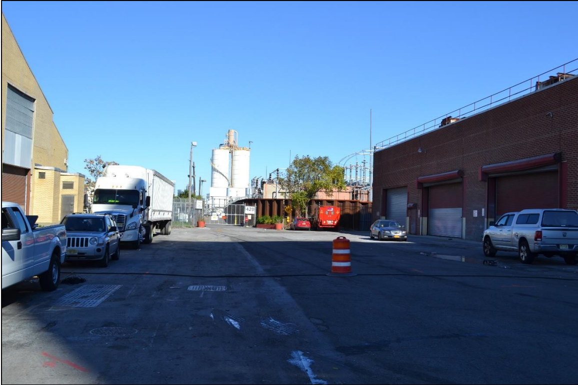
Photograph 1. Second Avenue and 29 th Street, Brooklyn, NY. View to northeast.
