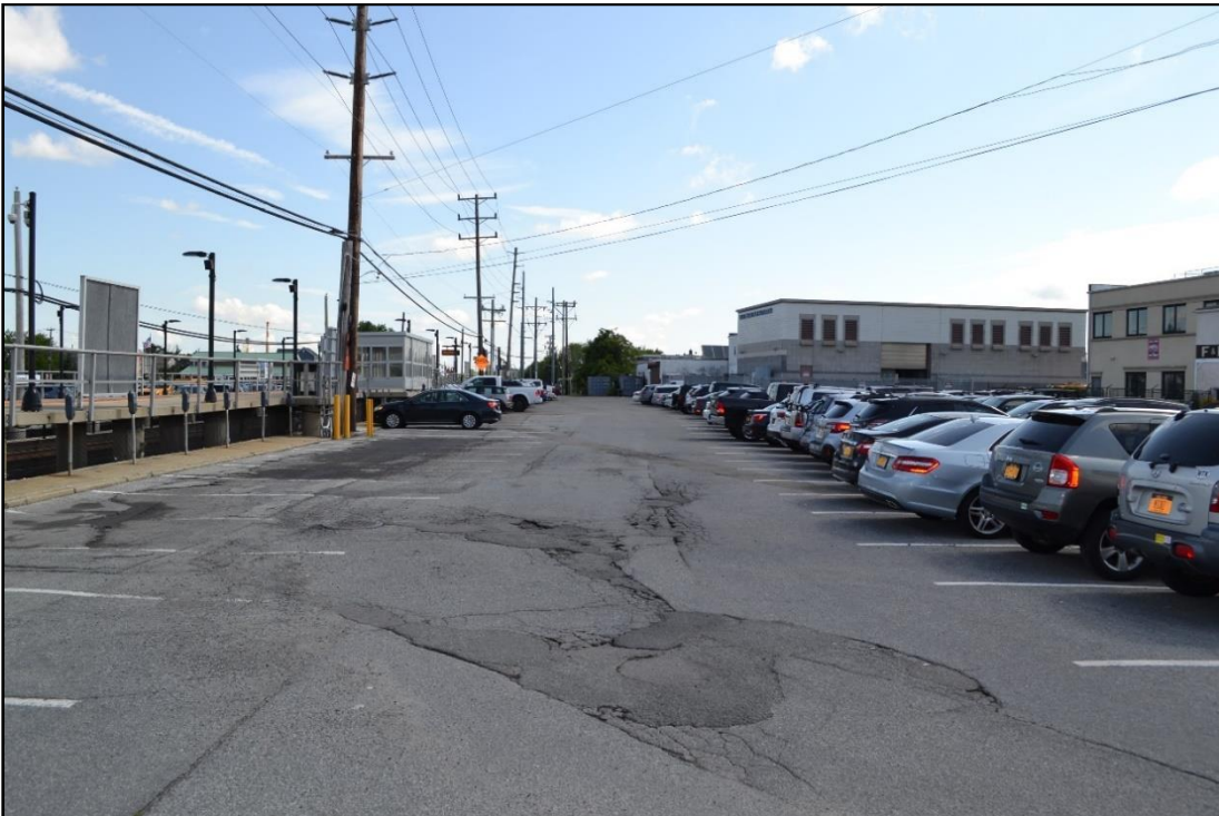
Photograph 2 EW 2 Route IP-C, LIRR Island Park Station. View to northeast.
