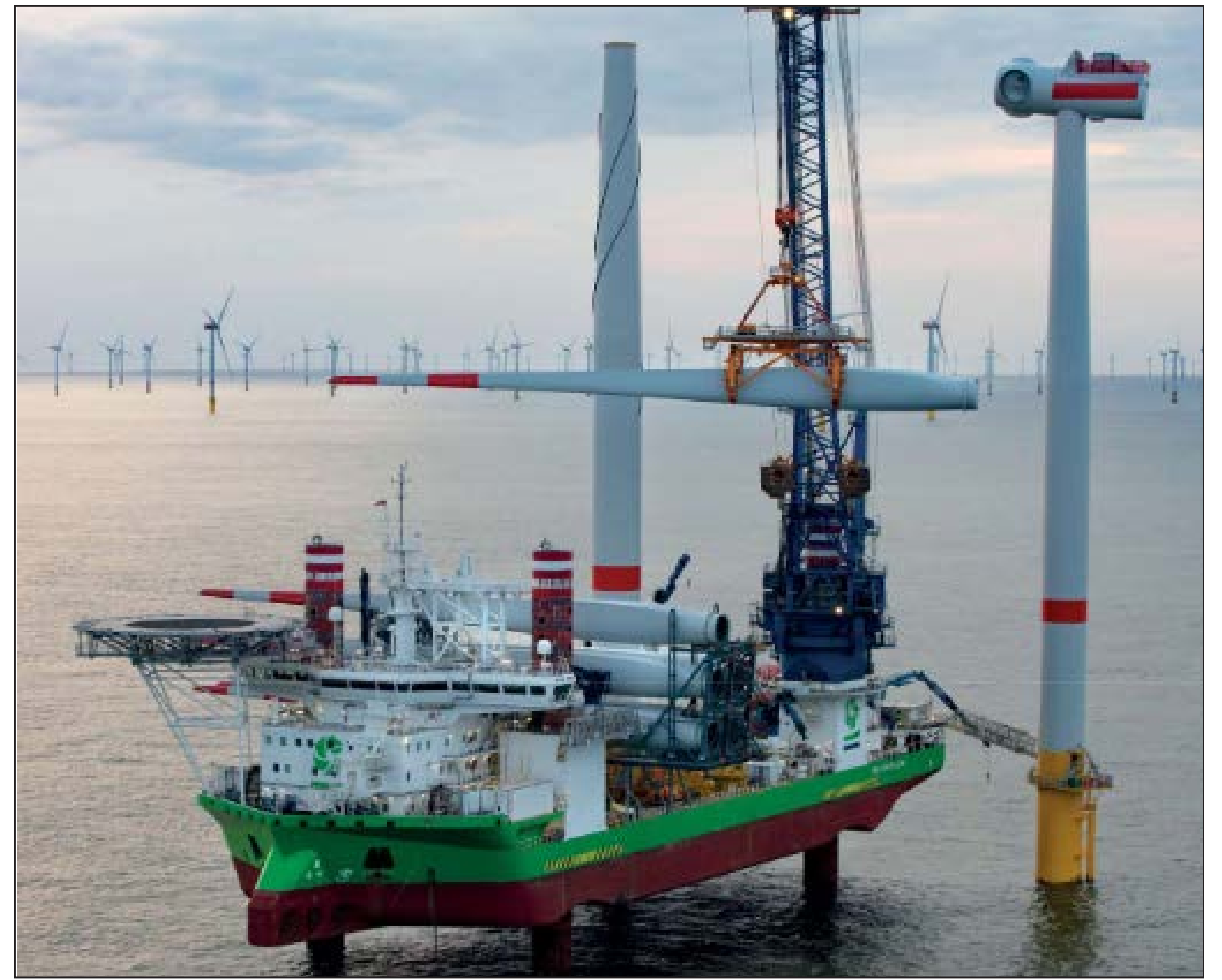
Installation of WTG Component using Jack-Up Vessel Crane
