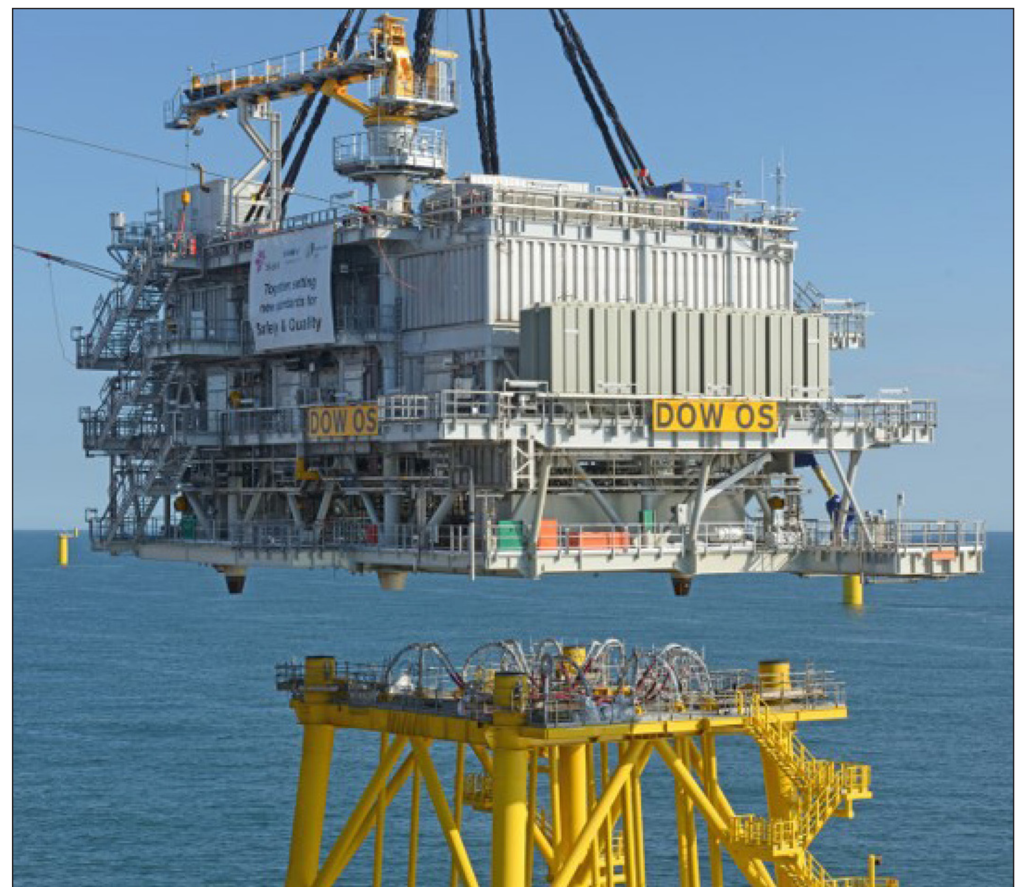
Installation of Offshore Substation
