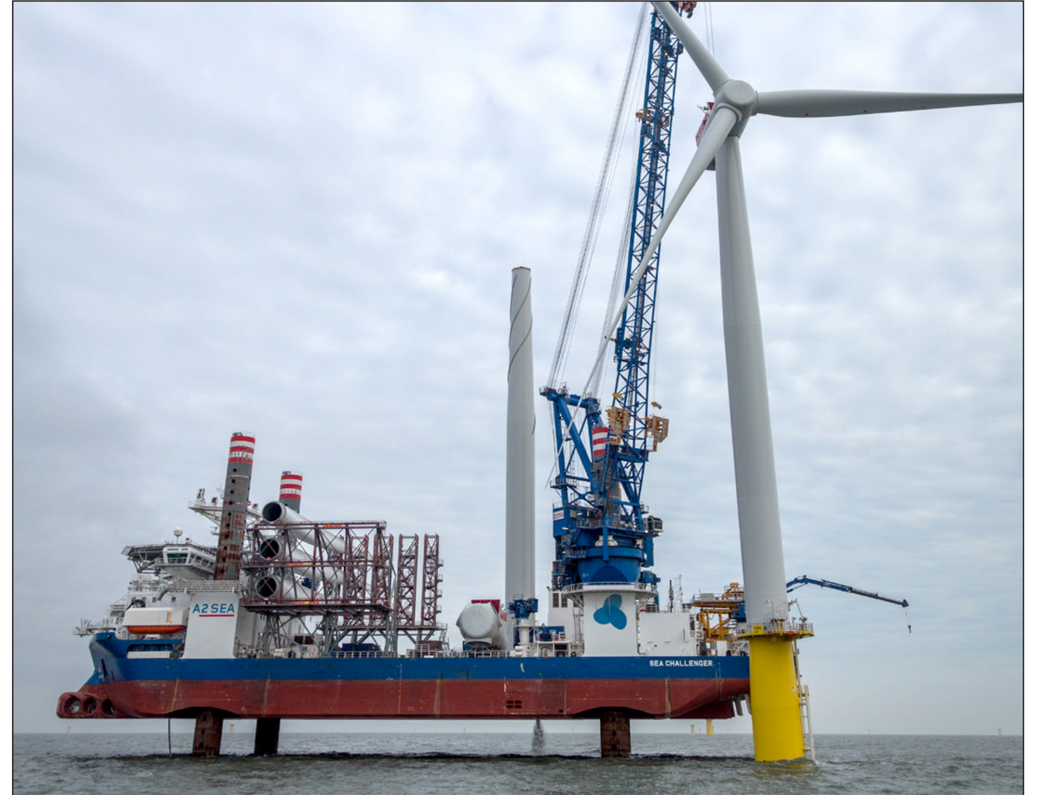
Wind Turbine Installation
