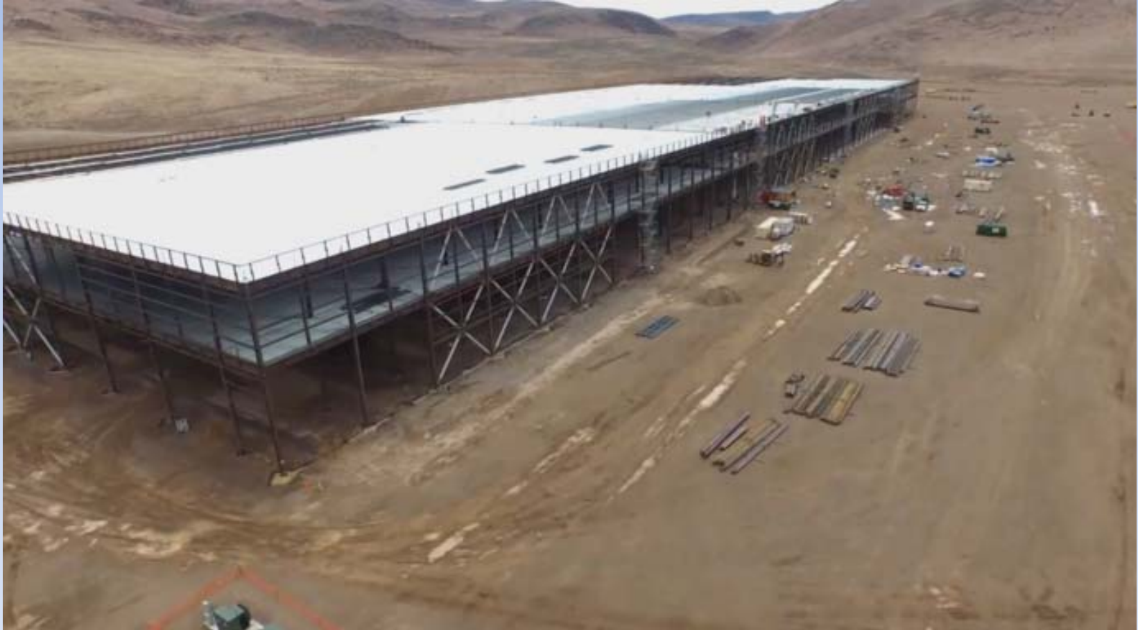
$5 B Tesla Battery Factory under construction
