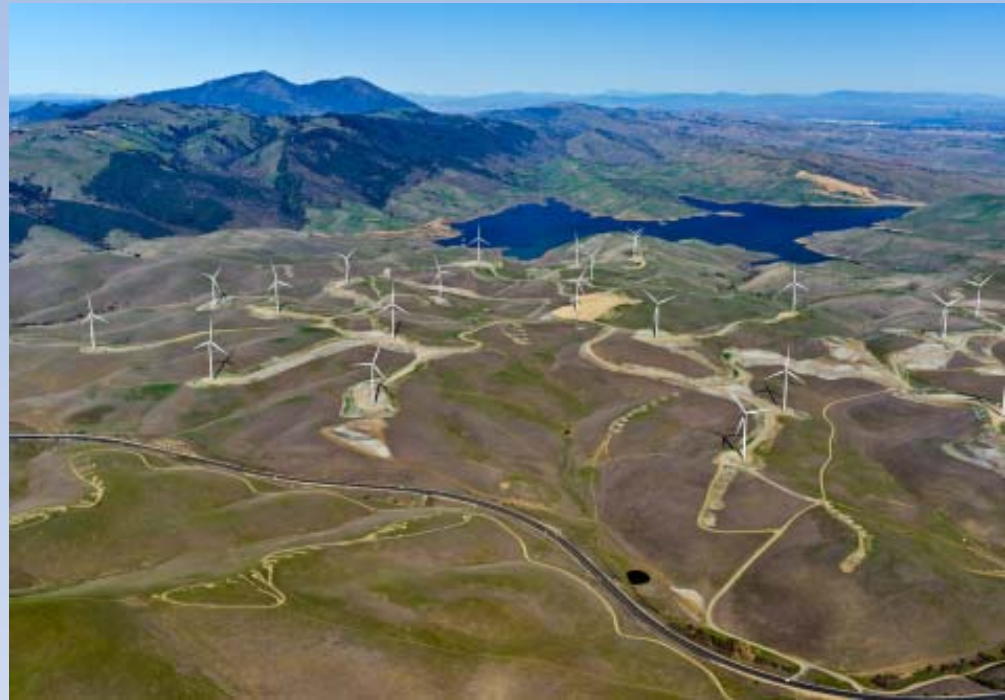
Vasco Wind Energy Center, 78MW Contra Costa County
