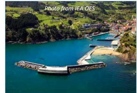
Photo from IEA OES European OWC Wave Power Plant, Azores
