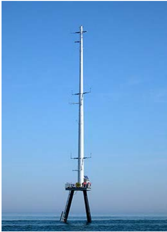
Figure 3-5 Example of Monopole-mast Meteorological Tower
