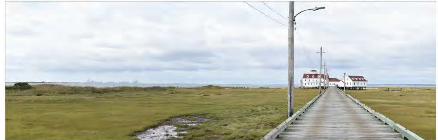
1. View looking southwest from access gate on boardwalk toward U.S. Coast Guard Station #119 (Rutgers Marine Field Station). Atlantic City skyline is visible on left side of image.
