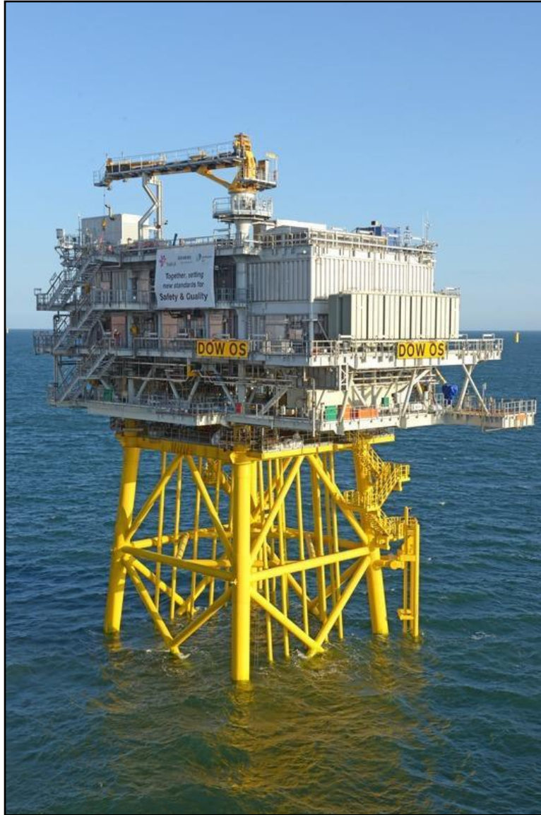
Figure 3.3-5 Example of an Offshore Substation on a Jacket Foundation (Equinor-operated Dudgeon Offshore Wind Farm)
