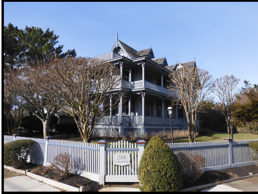
Sea Grove Historic District (MDWP-004), Ocean view, Maritime setting
