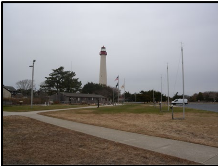
Cape May Lighthouse (7752), Ocean view, Maritime setting
