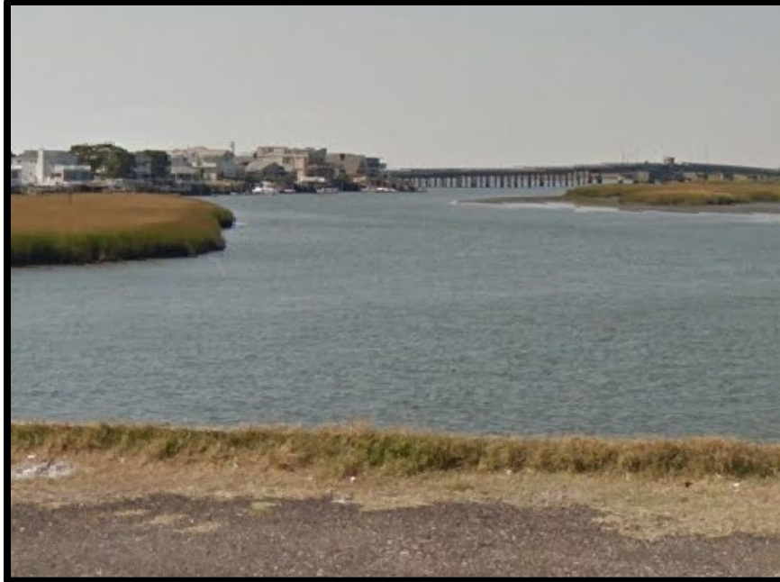
Ocean Highway Bridge (4763), No ocean view, Maritime setting
