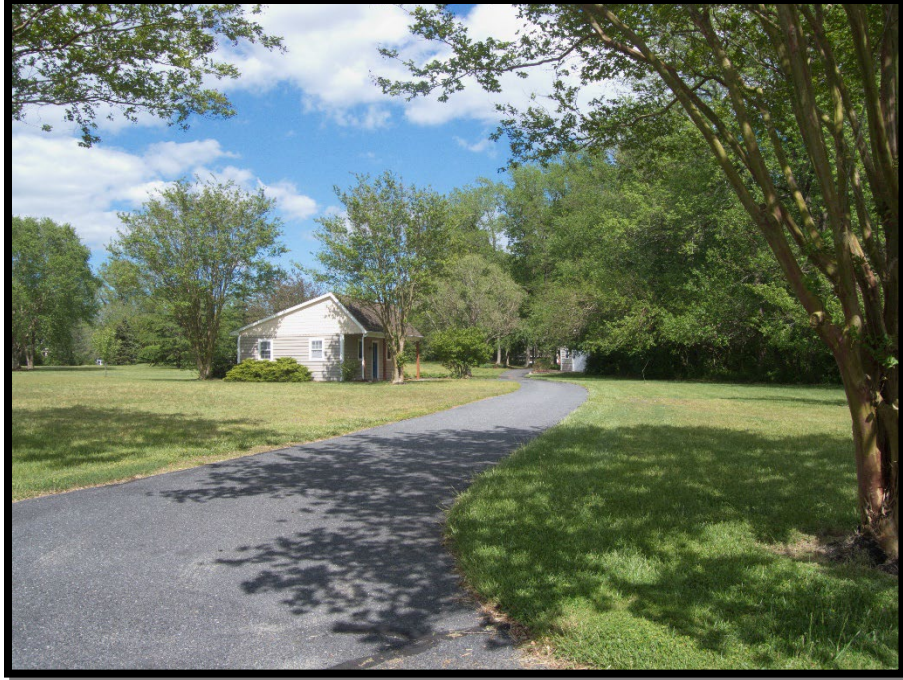
Fassitt House (WO-13), No ocean view, No maritime setting
