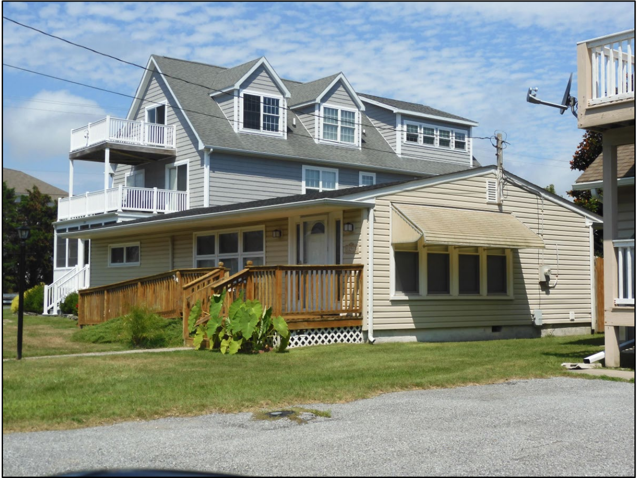
12915 Carmel Avenue façade and east elevation, facing northwest (RCG&A, August 2023)
