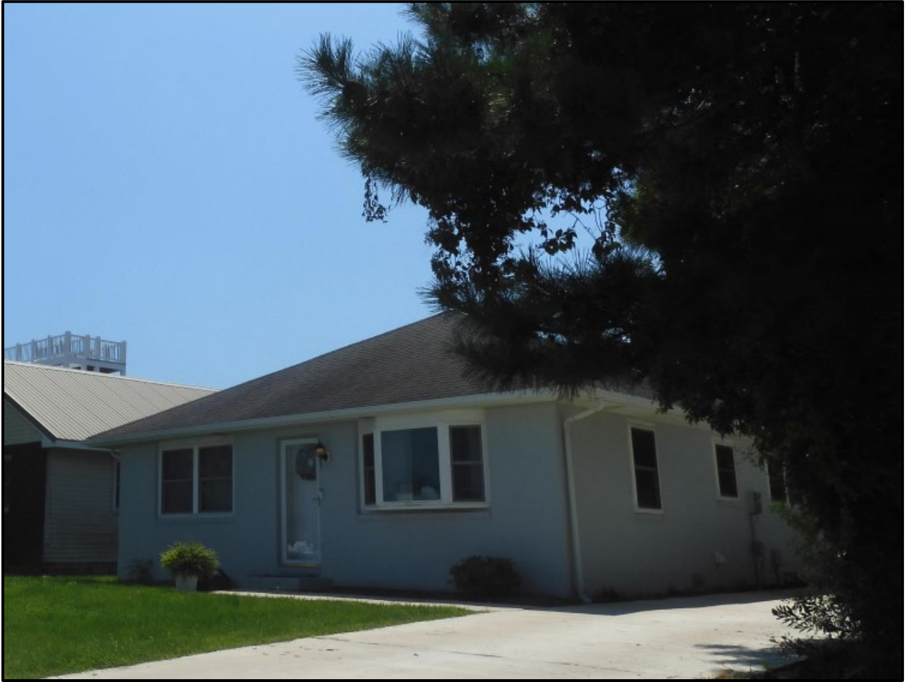
Building façade and west elevation, facing southeast (RCG&A, August 2023)
