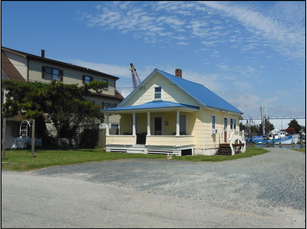
12849 Harbor Road façade and east elevation, facing northwest (RCG&A, August 2023)
