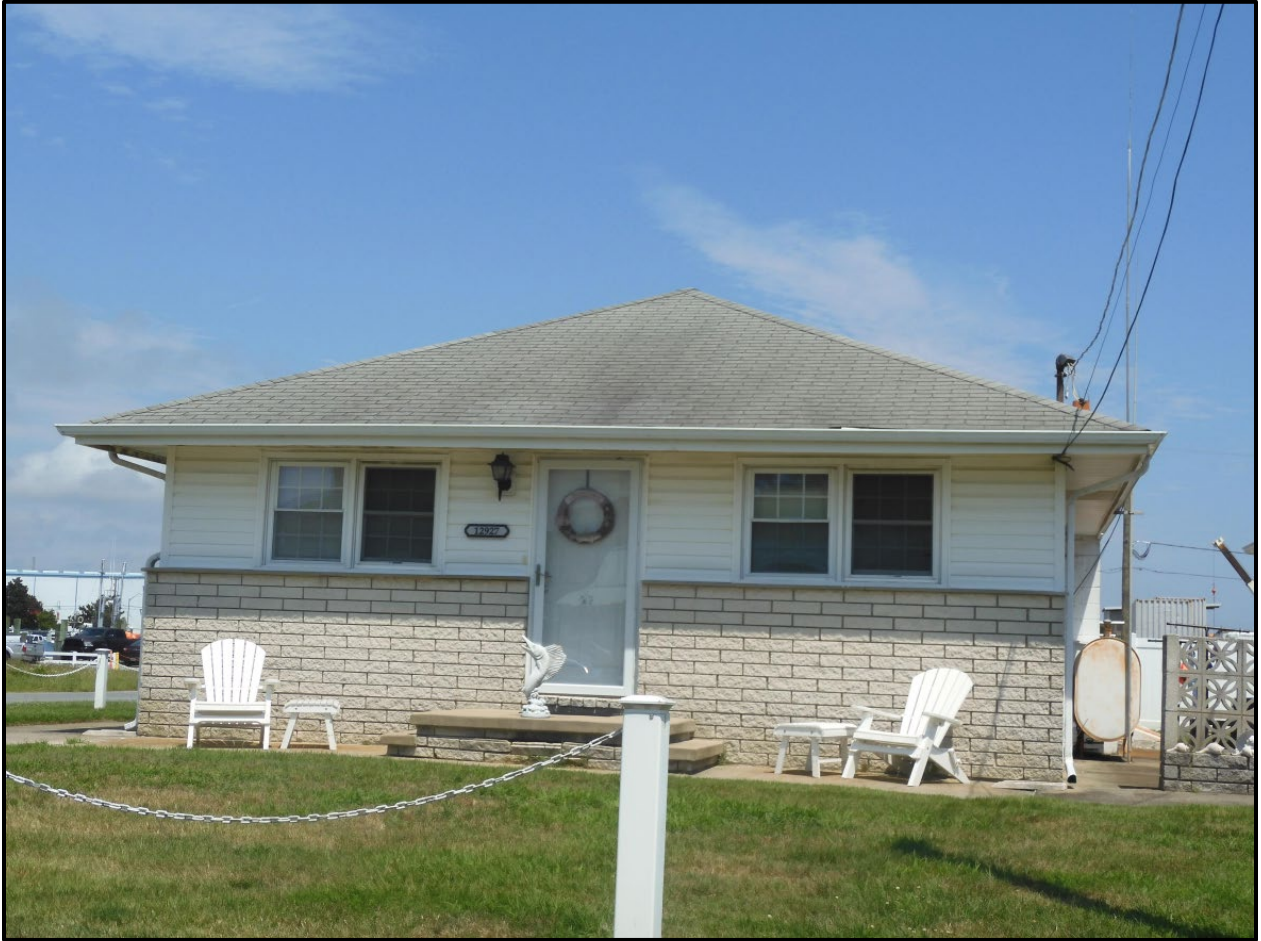
12927 Swordfish Drive façade facing north (RCG&A, August 2023)
