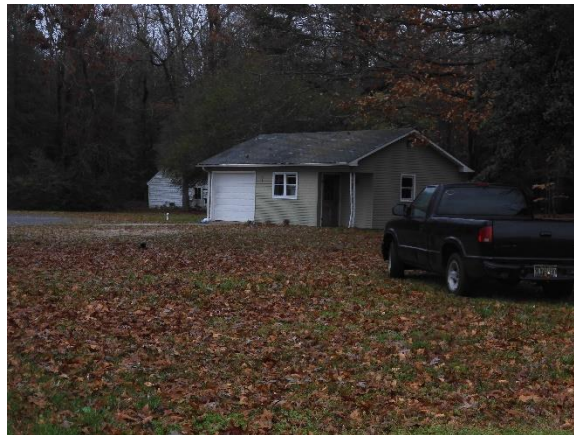
Garage outbuilding façade and southeast elevation, facing north
