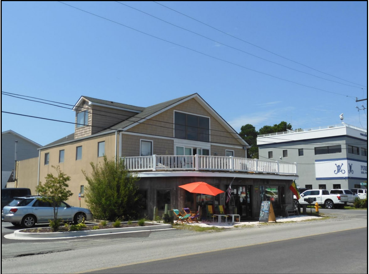
12814 Harbor Road façade and east elevation, facing southwest (RCG&A, August 2023)
