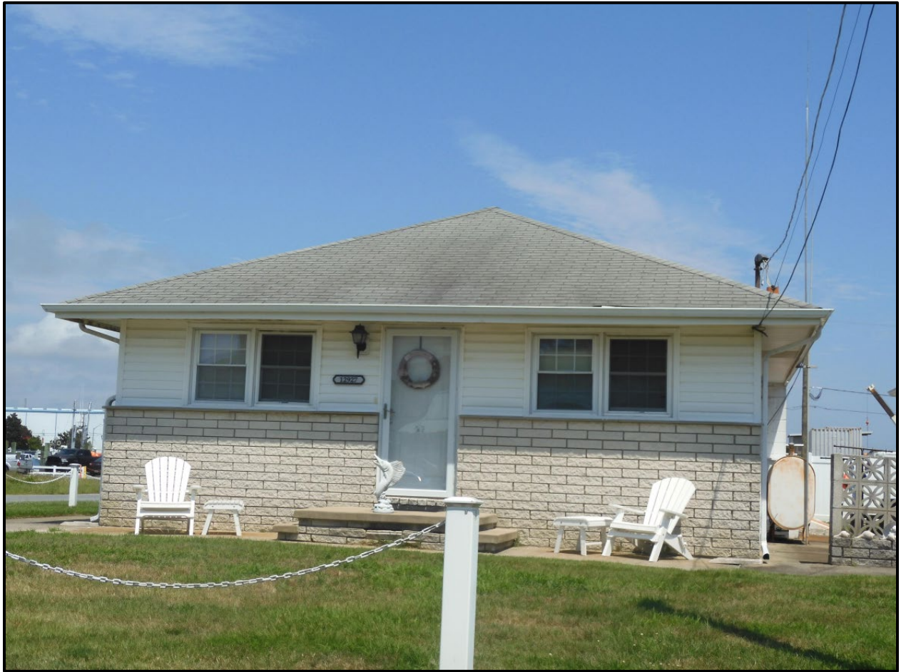
12927 Swordfish Drive façade facing north (RCG&A, August 2023)
