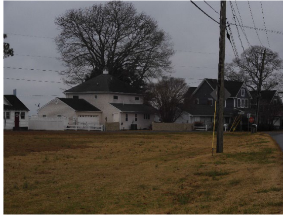
28828 Point View Road façade and south elevation, facing northwest
