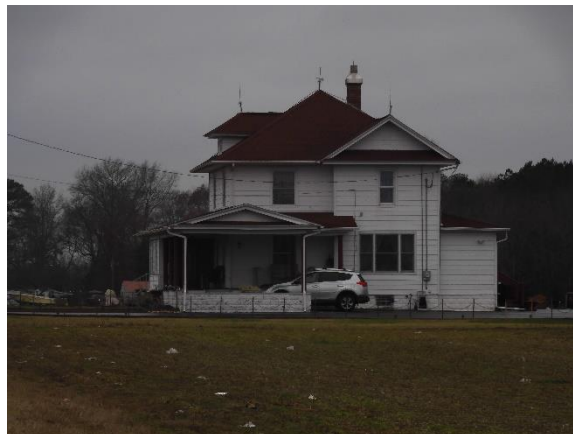
28808 John J. Williams Highway east elevation, facing west
