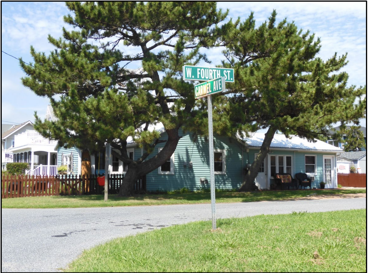
9623 W 4 th Street façade and east elevation, facing northwest (RCG&A, August 2023)
