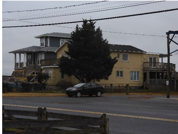
32150 River Road, Façade and north elevation facing southwest
