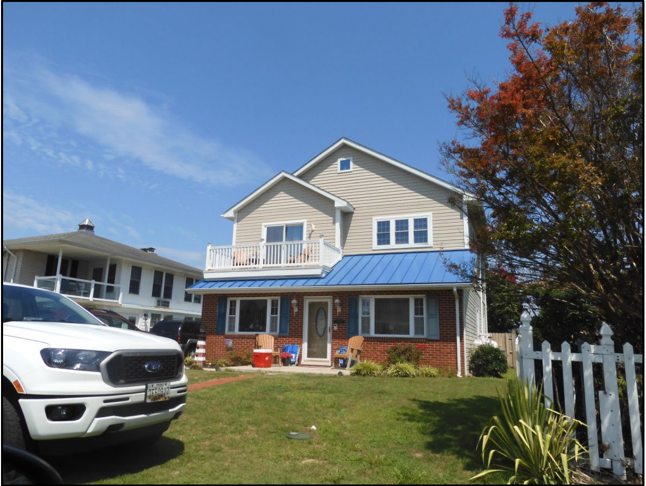
12939 Swordfish Drive façade, facing northwest (RCG&A, August 2023)
