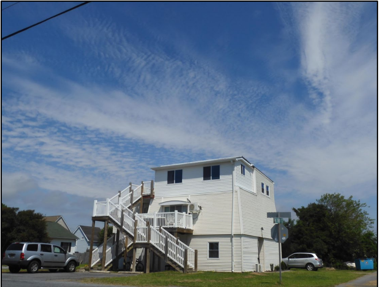
12905 Swordfish Drive façade and east elevation, facing northwest (RCG&A, August 2023)
