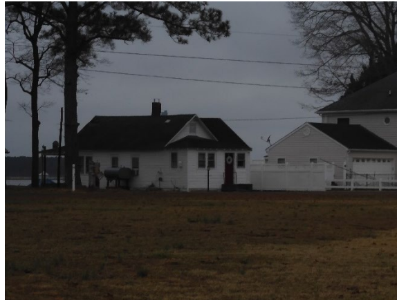
28830 Point View Road, Façade and south elevation facing northwest
