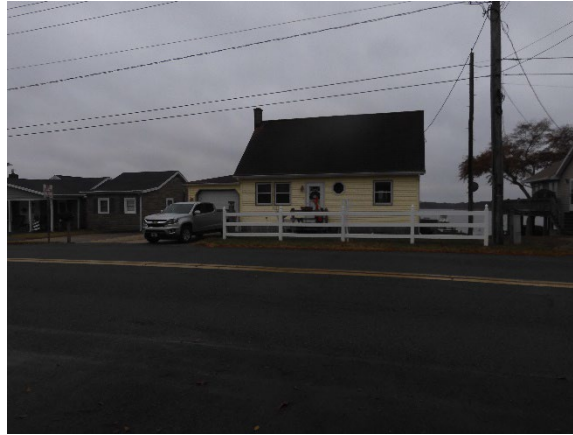
31457 River Road façade, facing west.
