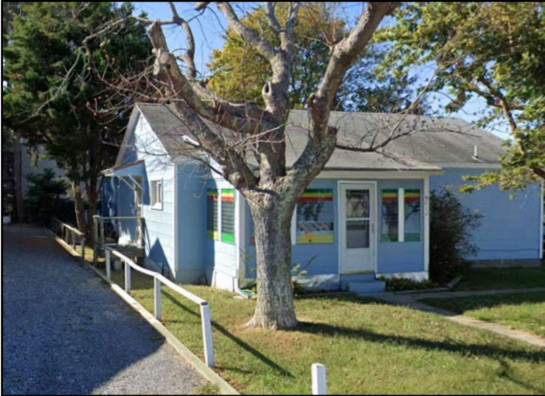
9643 Harbor Road façade and south elevation, facing northwest (Google, 2019) 2
