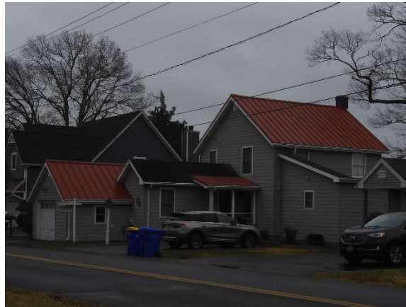
31490 River Road façade and north elevation, facing southwest.
