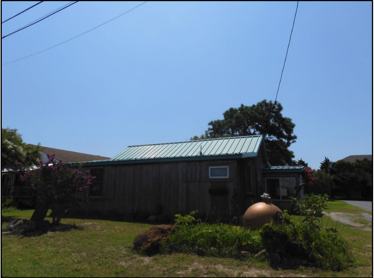
12928 Swordfish Drive north elevation, facing south (RCG&A, August 2023)
