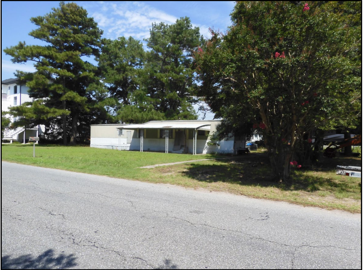
12823 Swordfish Drive façade and east elevation, facing northwest (RCG&A, August 2023)
