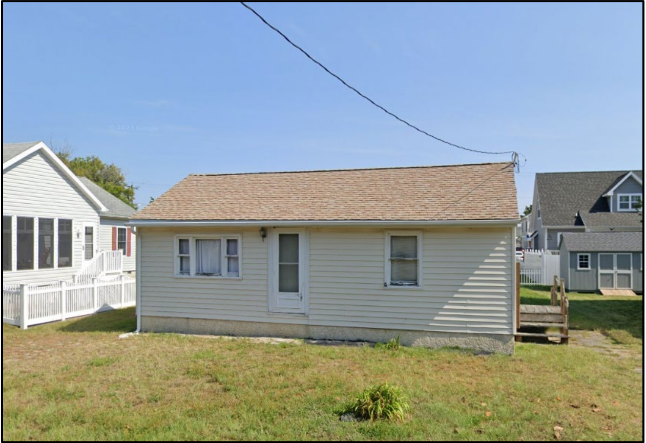
12935 Carmel Avenue façade, facing north (RCG&A, August 2023)
