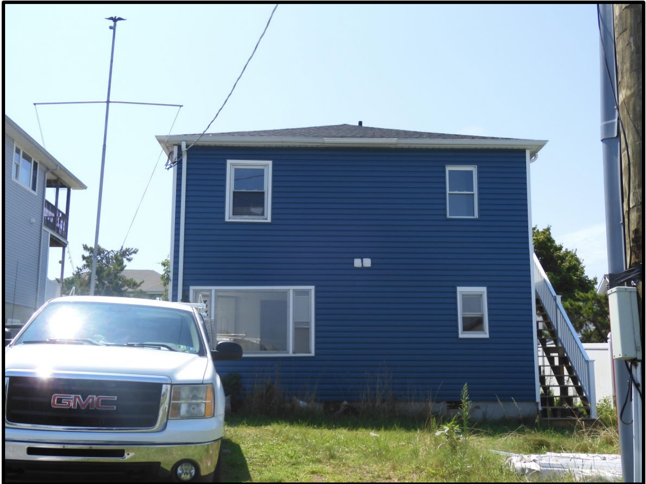
12924 Swordfish Drive façade, facing south (RCG&A, August 2023)
