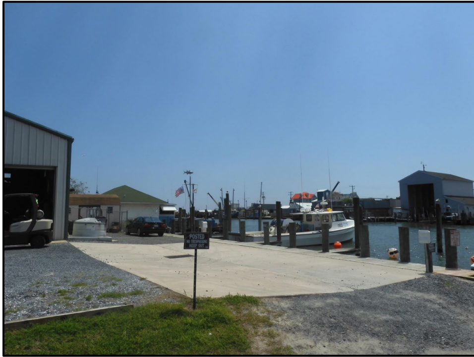
Figure 2.13. Commercial development at the harbor looking southeast toward the proposed O&M Facility site (RCG&A 2023)
