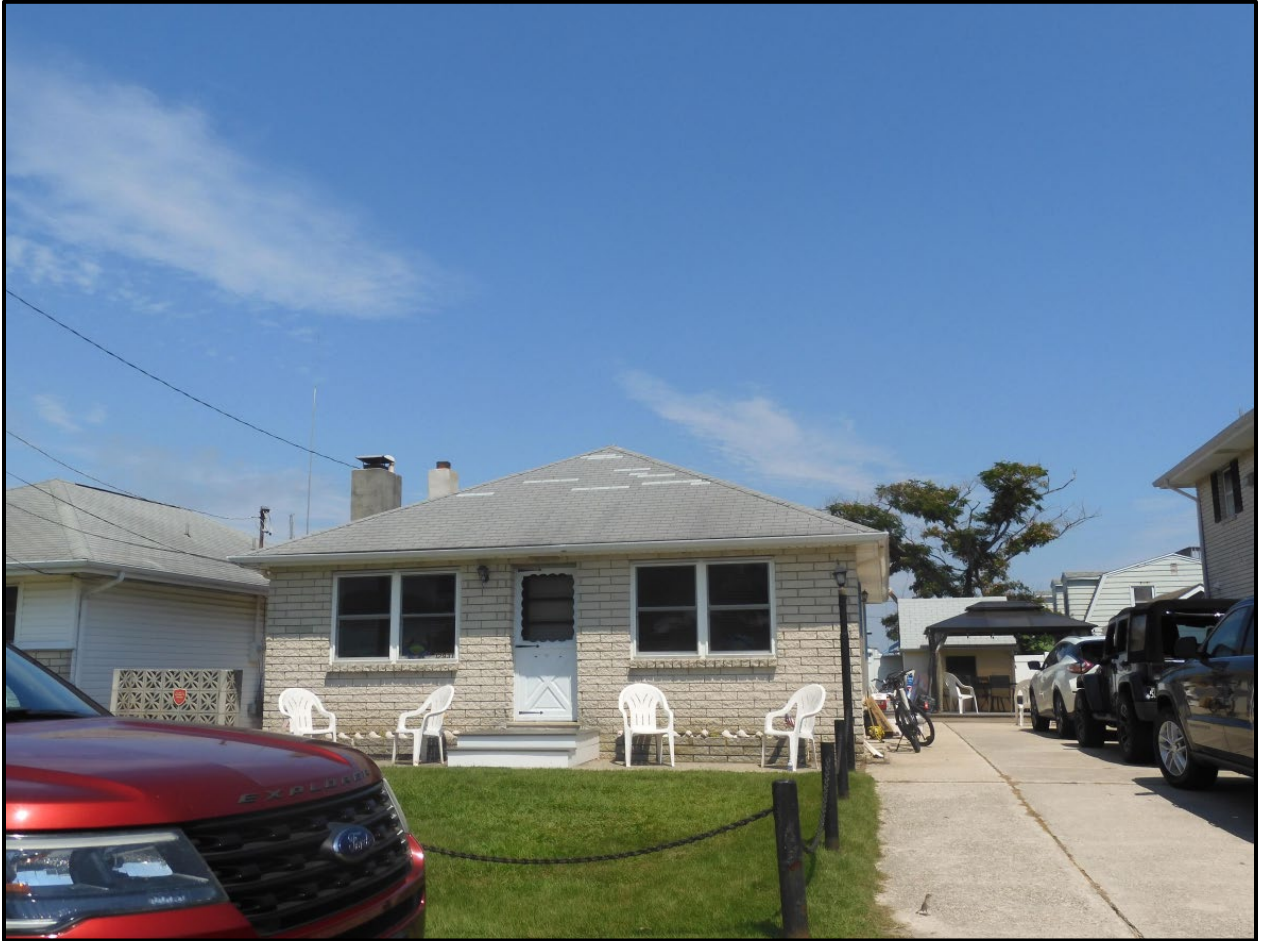
12931 Swordfish Drive façade facing north (RCG&A, August 2023)
