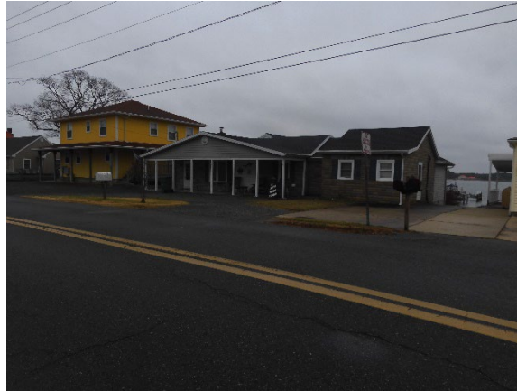
31470 River Road façade and north elevation, facing southwest.
