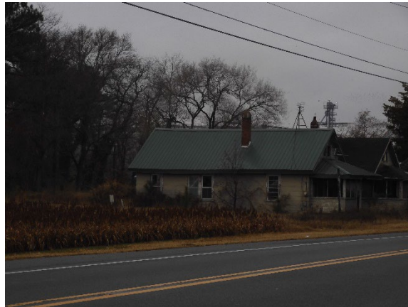
28925 John J. Williams Highway detail, facing southwest
