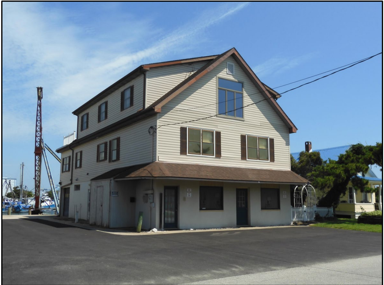
12845 Harbor Drive façade and west elevation, facing northeast (RCG&A, August 2023)
