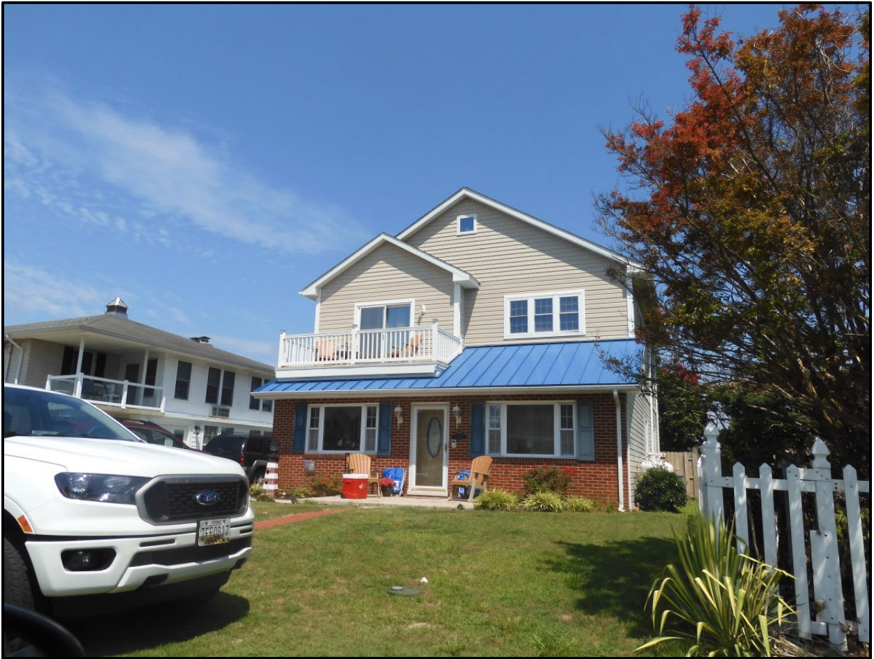
12939 Swordfish Drive façade, facing northwest (RCG&A, August 2023)
