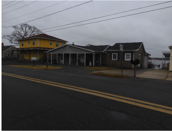
31470 River Road façade and north elevation, facing southwest.
