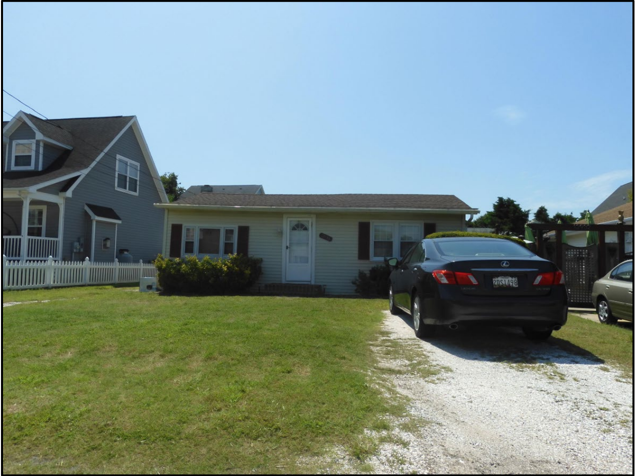
12936 Swordfish Drive façade facing south (RCG&A, August 2023)
