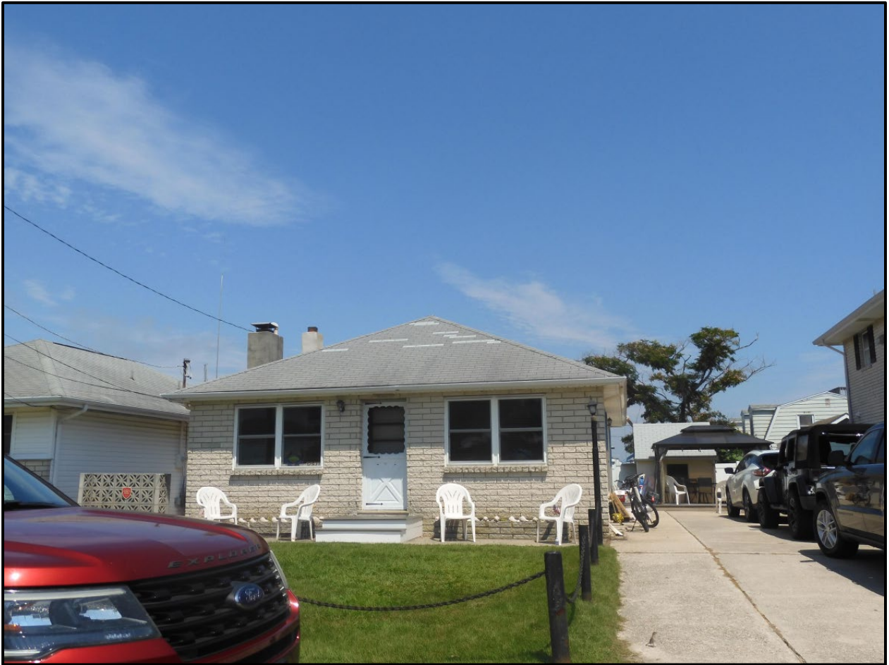
12931 Swordfish Drive façade facing north (RCG&A, August 2023)
