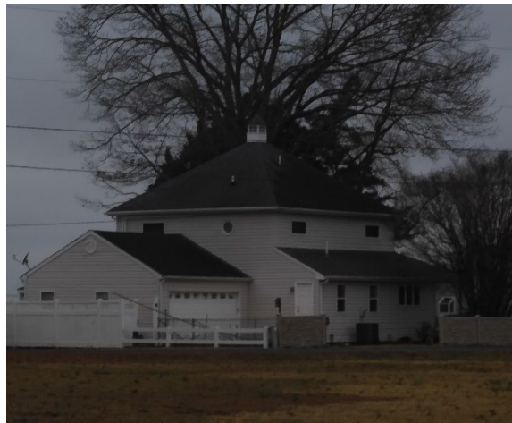
28828 Point View Road detail, facing northwest
