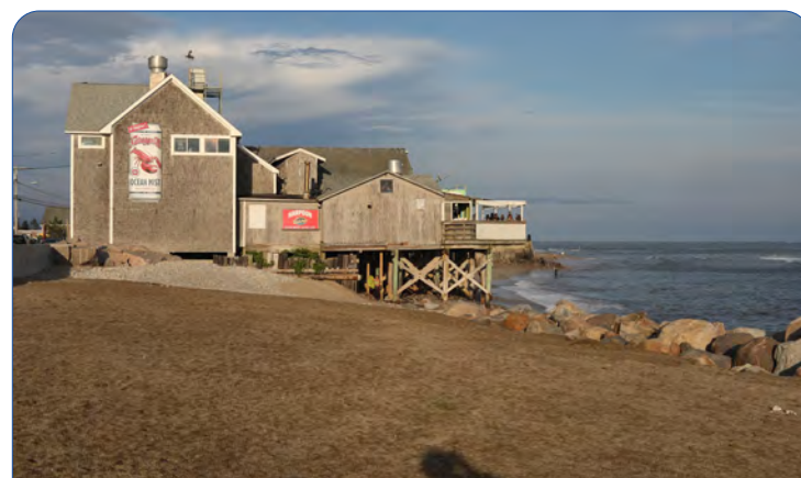
Context Photo: View to the East
