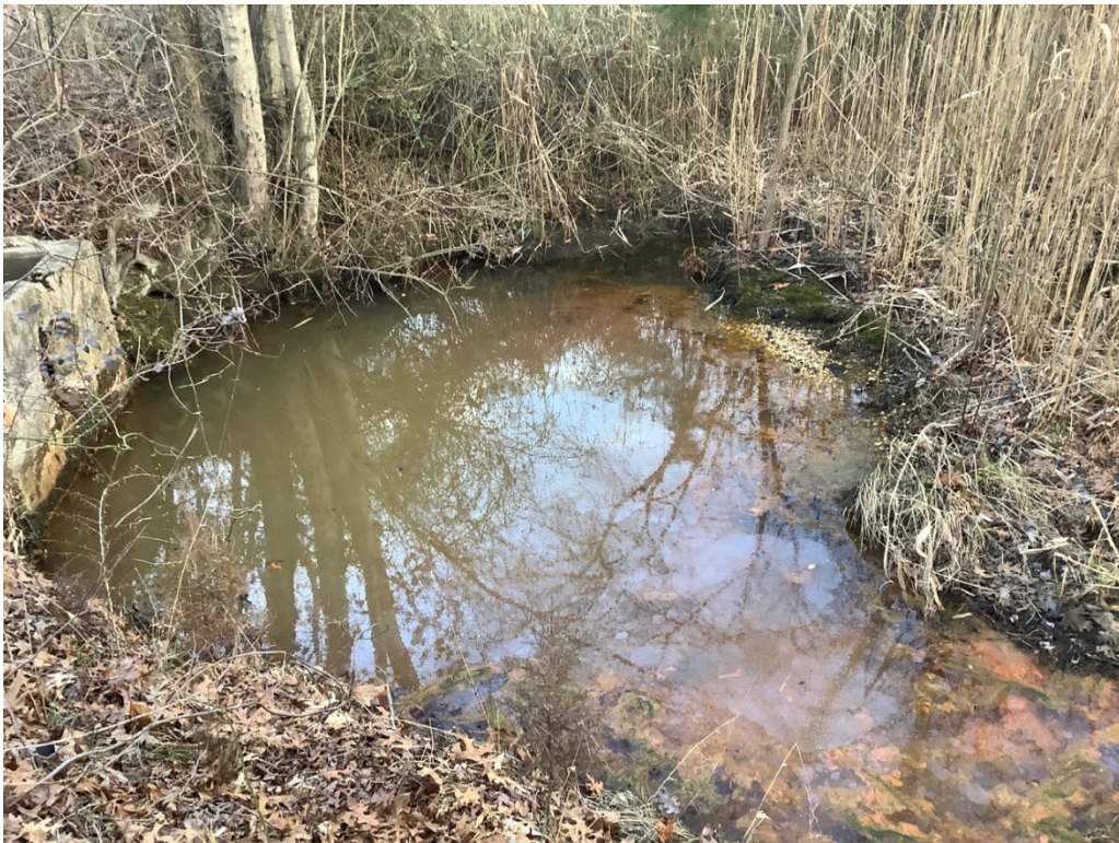
Photograph 2. Pool of water created by wetland and culvert
