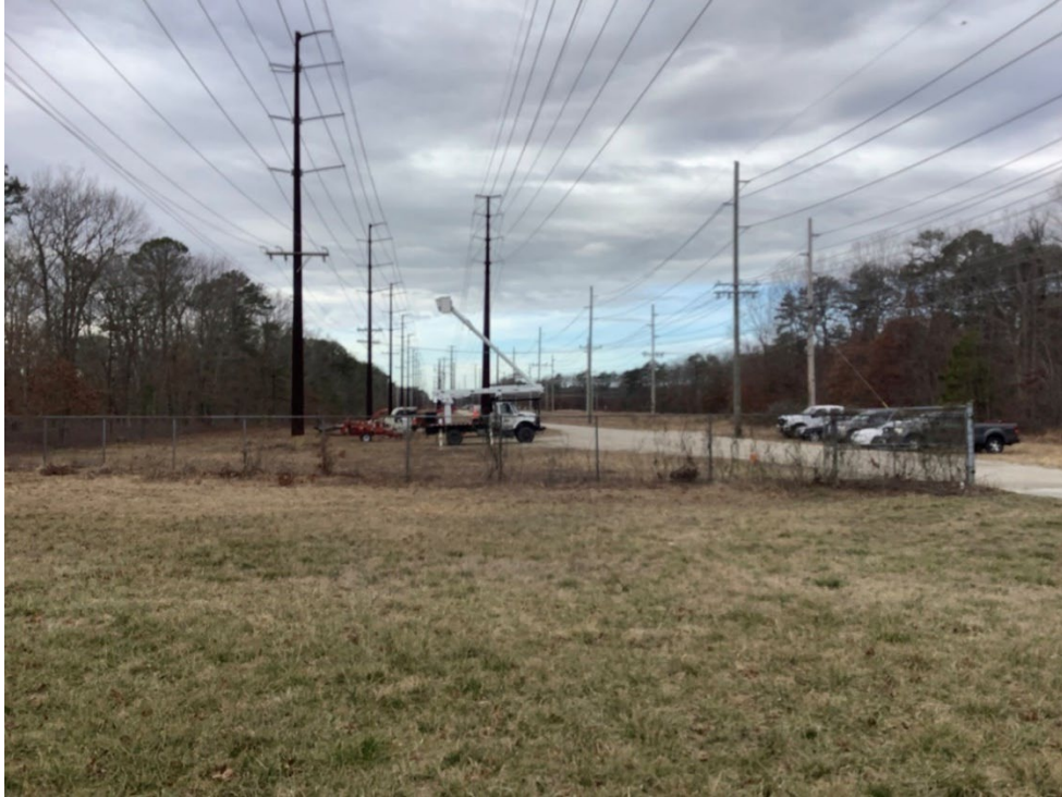
Photograph 3. Representative photograph of the current habitat east side of the Cardiff Substation along English Creek Avenue consisting of mowed lawn to the east of the Substation
