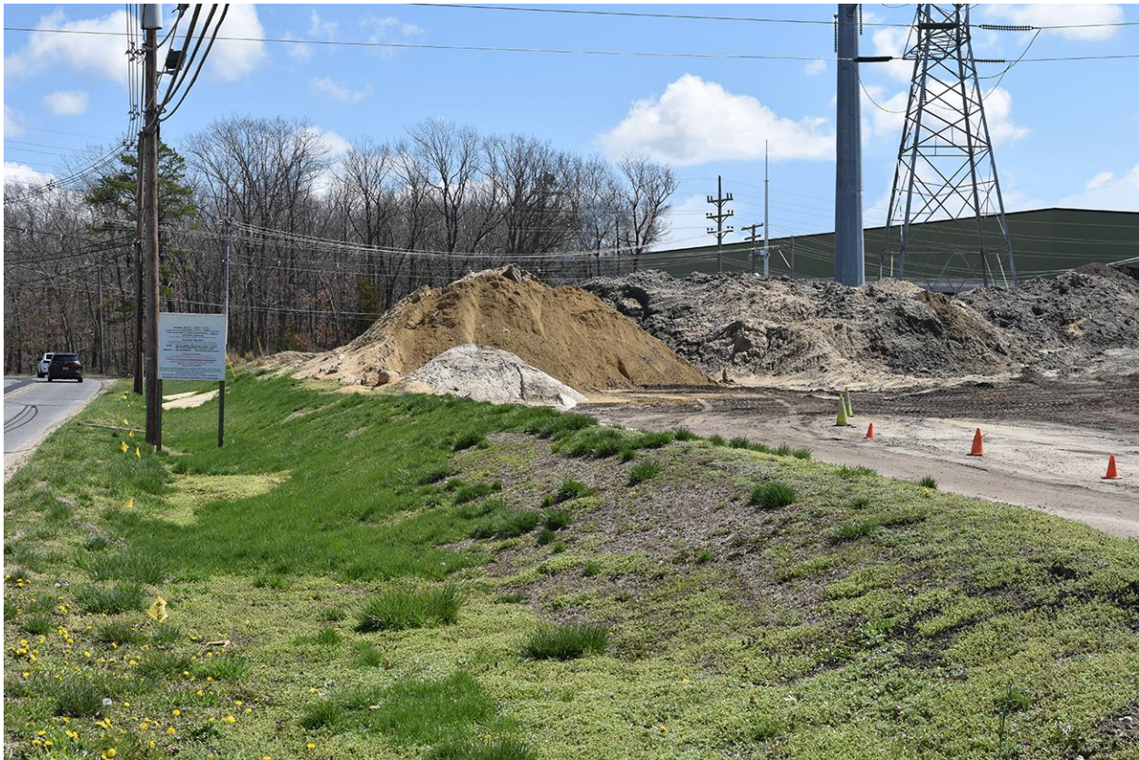
Inset 2.3-10. Brook Road Substation/Converter Station with mitigation from KOP 5 on Randolph Road
