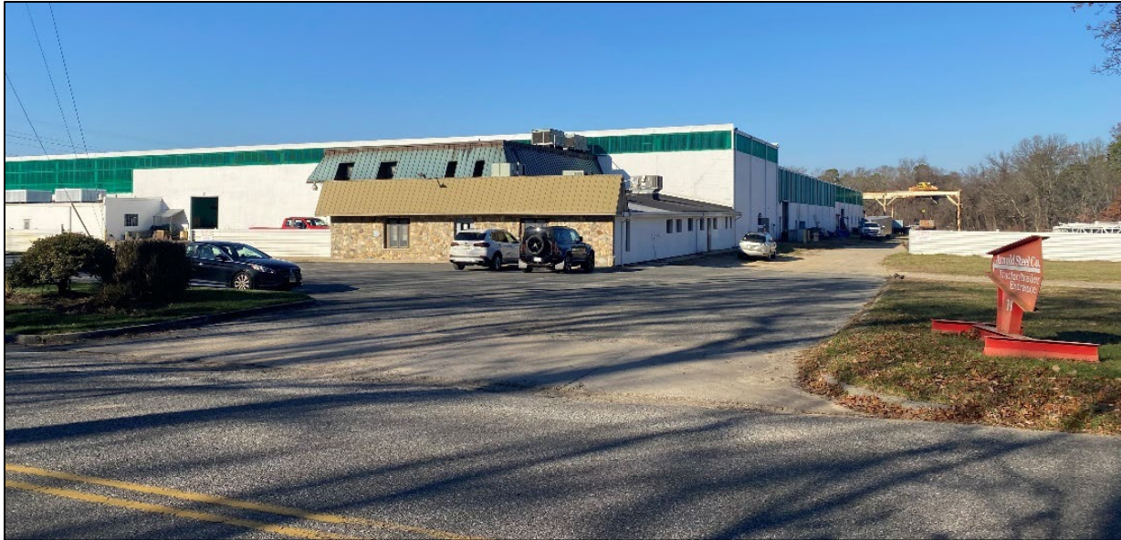
Figure 2.1-3. The Randolph Road Site overview. View of the steel fabricator facility from Randolph Road. View to the north.
