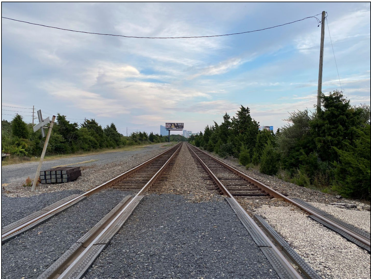
Figure 5.2-7. The West Jersey and Atlantic Railroad Historic District
