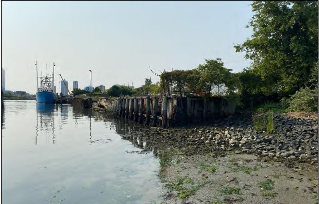
Photograph 3. Overview of partially collapsed wood and concrete bulkhead facing the marina. View to the south.
