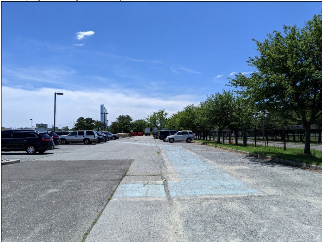
Figure 2.2-5. Overview of the state marina parking lot parcel, showing the fencing and perimeter landscaping bordering North Maryland Avenue, view to the south.
