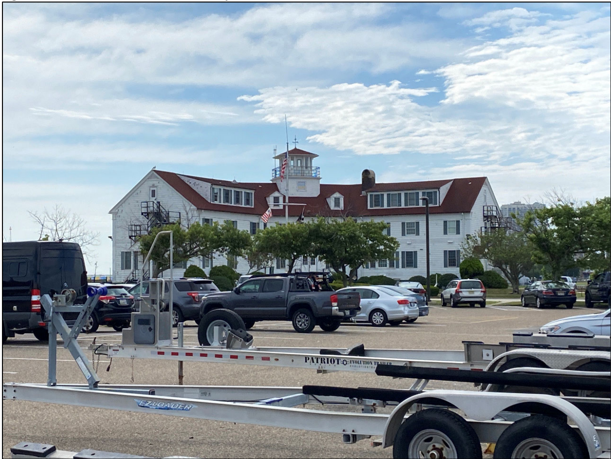
Figure 5.2-7. USCG Station Atlantic City.
