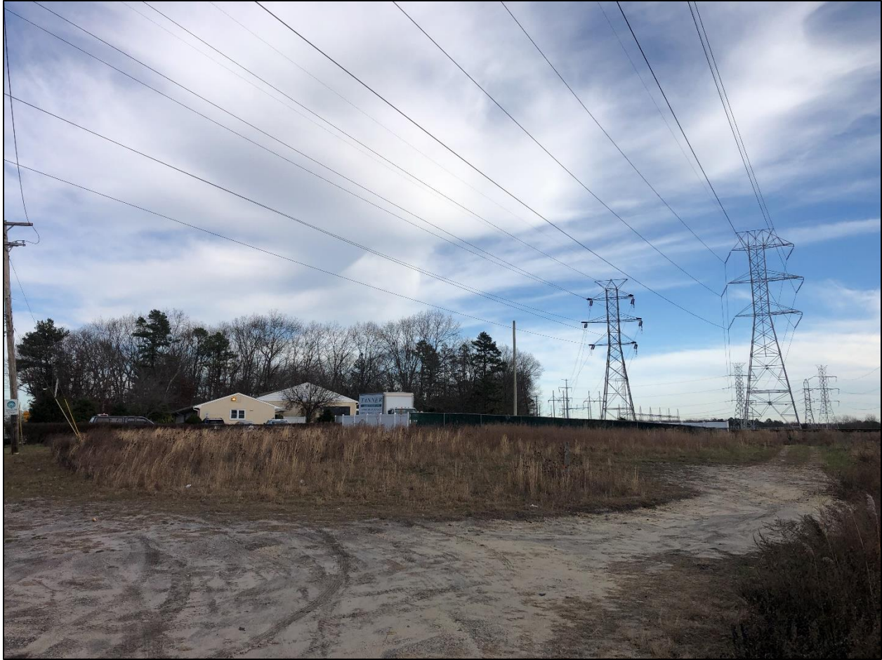
Figure 3.2-1 View to the north-northeast toward the proposed substation Site.
