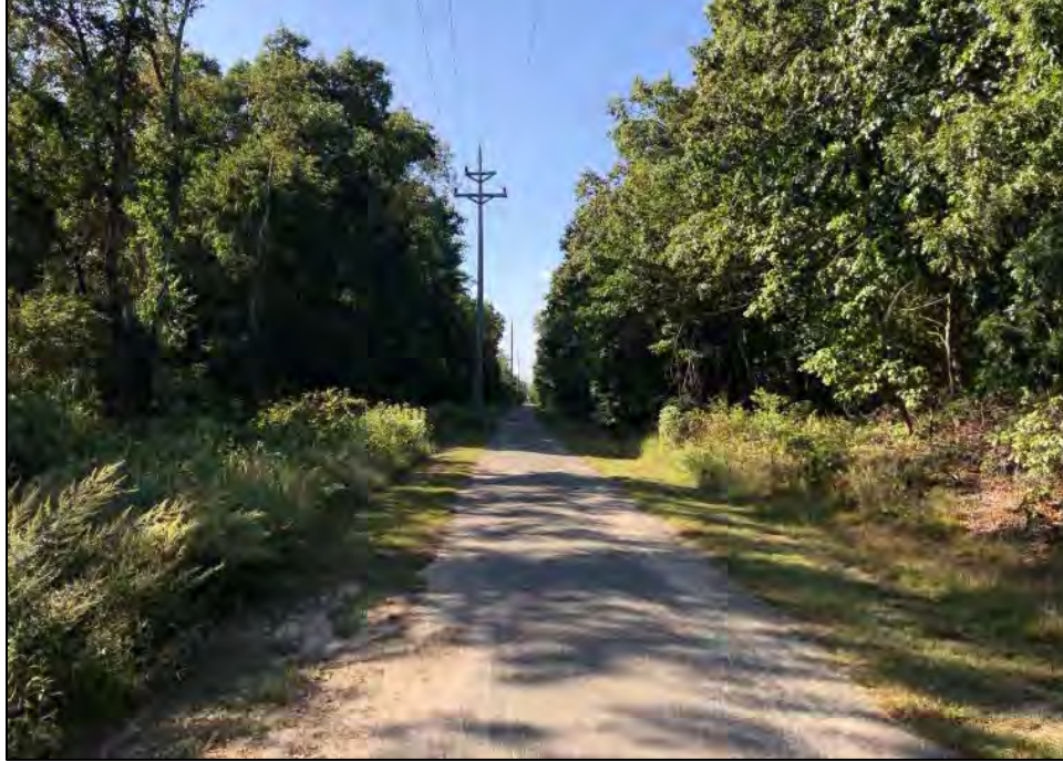
Photograph 6. Area of Larrabee Onshore Route along Edgar Felix Memorial Bikeway, west of NJ Route 34. Note the overhead transmission line. View to the northwest.
