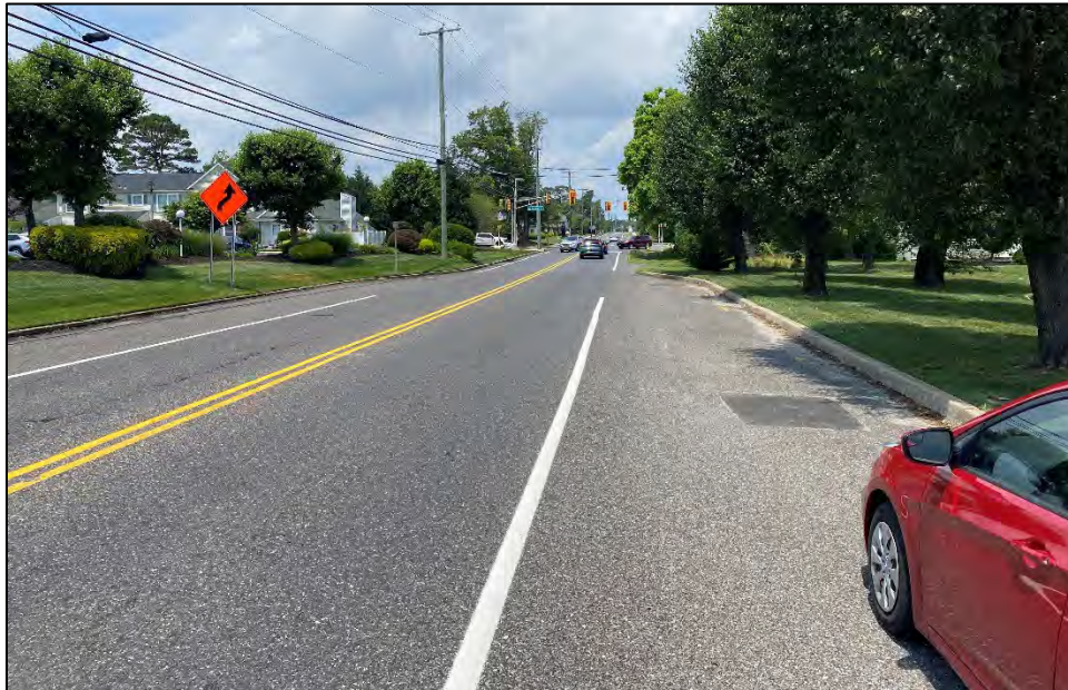
Photograph 28. Overview of the Cardiff Onshore Route option along old Egg Harbor Road, leading to the Fire Road Site substation location. View to the northwest.
