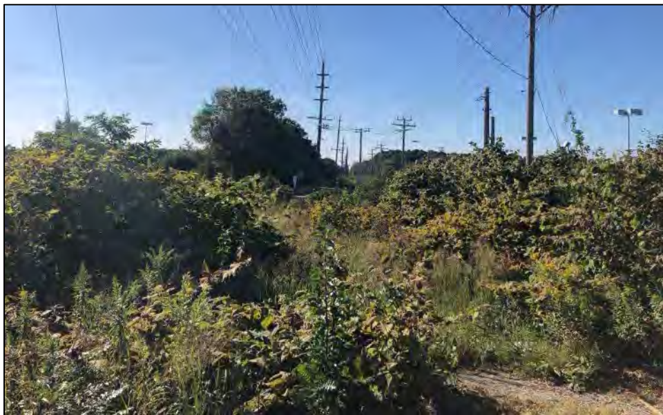
Photograph 29. Overview of the Cardiff Onshore Route west of the Garden State in overgrown ACE and inactive railroad ROW. View to the northwest.
