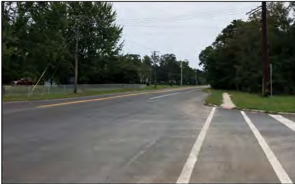
Photograph 31. Overview of the Cardiff Onshore Route along east side of English Creek Avenue. View to the north.
