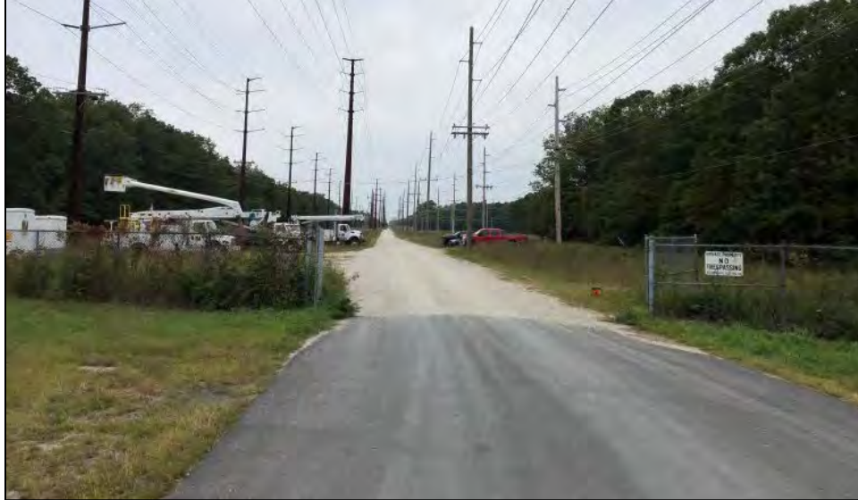
Photograph 32. Overview of the Cardiff Onshore Route at the interconnection of the existing high-tension ACE transmission corridor at the Cardiff POI. View to the west.
