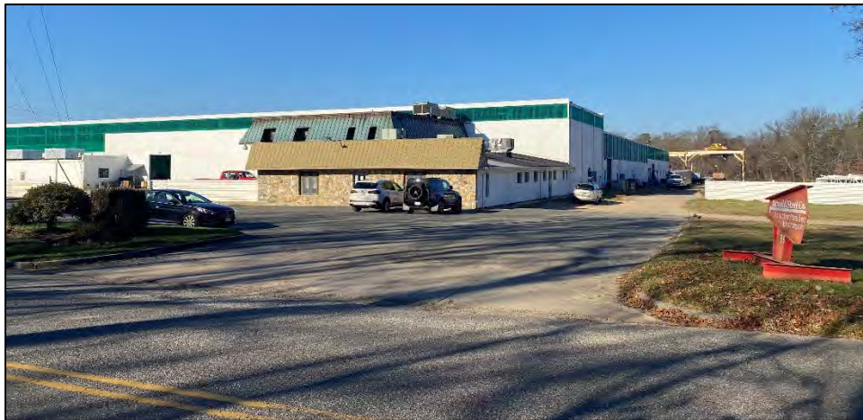
Photograph 18. The Randolph Road Site overview. View of the steel fabricator facility from Randolph Road. View to the north.
