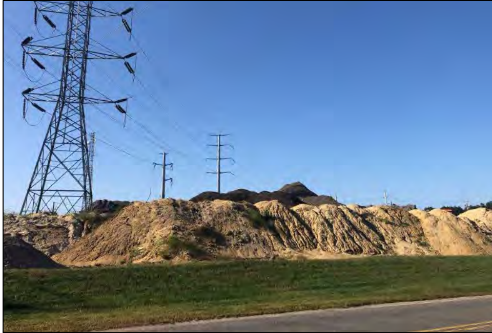
Photograph 13. Large push piles, bulk material storage, and pervasive ground disturbance on a parcel just north of the existing Larrabee POI. Note transmission towers leading to existing facility. View to the south.
