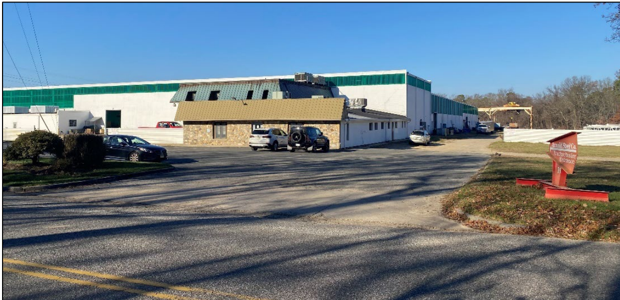
Figure 3.2-3. The Randolph Road option overview. View of the steel fabricator facility from Randolph Road. View to the north.
