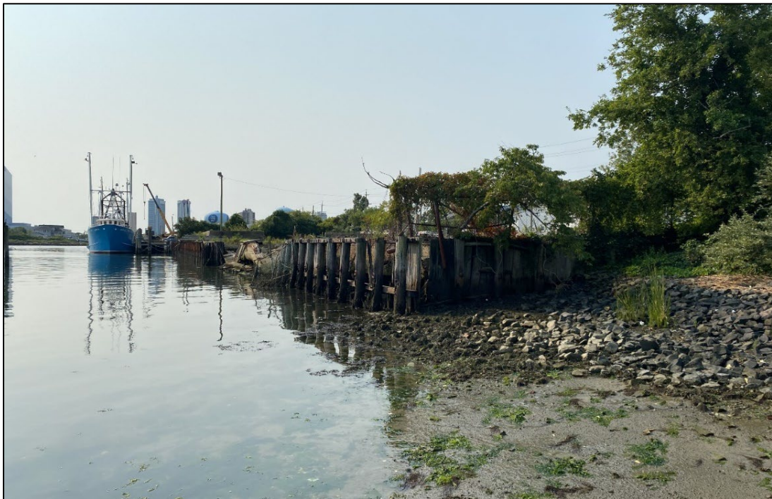
Figure 3.3-3. Overview of partially collapsed wood and concrete bulkhead facing the marina. View to the south.
