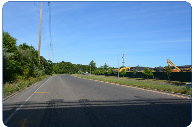
Viewpoint 4 - View from Long Island Ave, Town of Brookhaven, Suffolk County, looking Northwest
