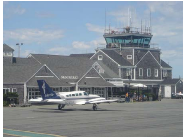
Figure 5-26. Light Industrial, Nantucket Memorial Airport
