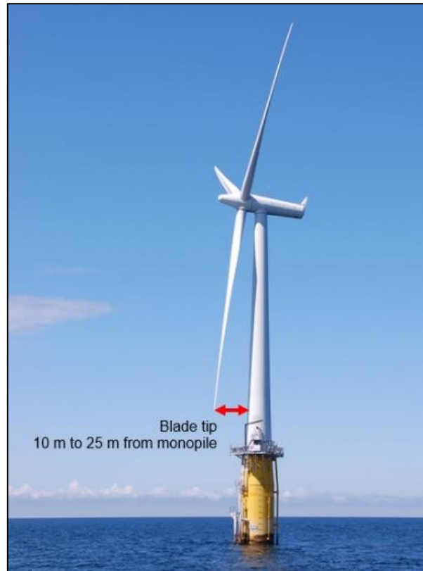
Figure 3-2 Illustration of blade tip distance from monopile
