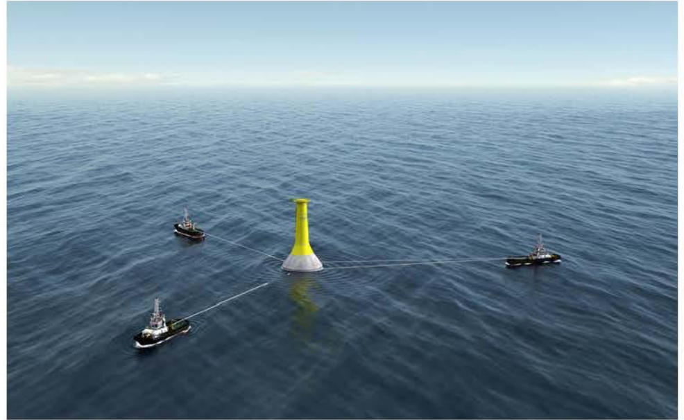
Gravity Foundation Transport via Tugboats
