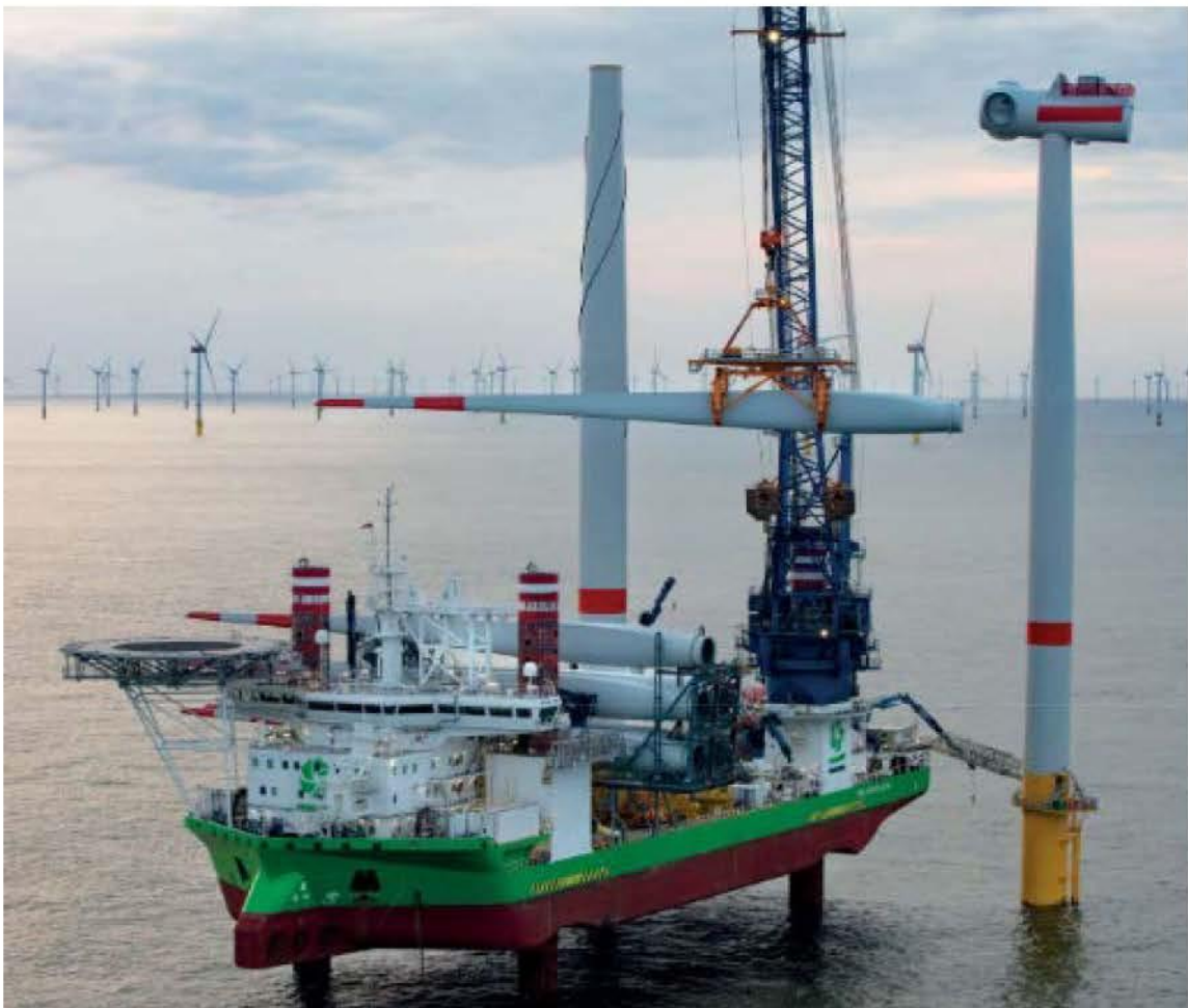
Installation of WTG Component using Jack-Up Vessel Crane
