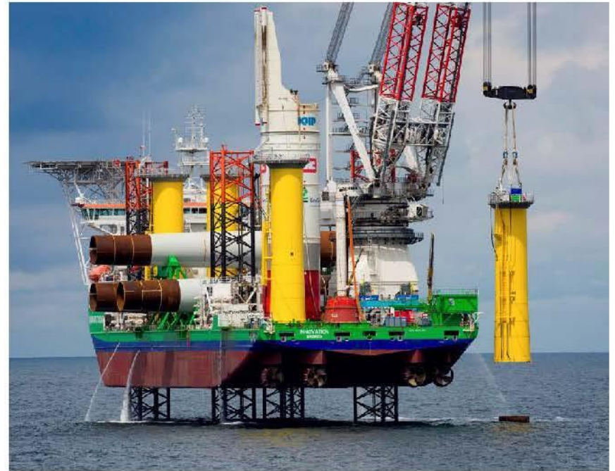
Transition Piece Installation from a Jack-Up Vessel
