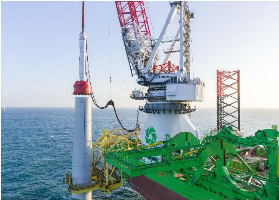
Pile Driving of a Monopile
