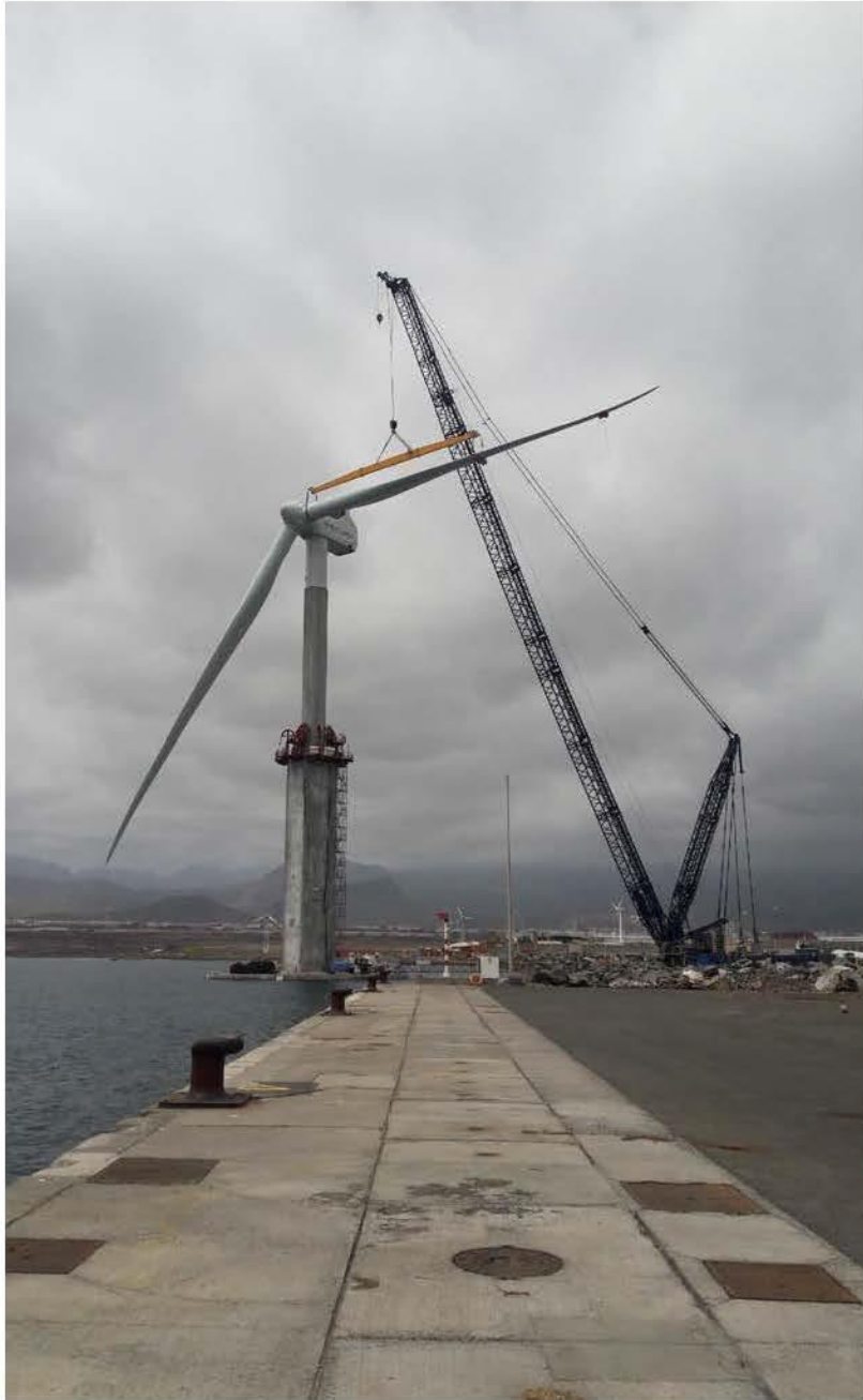
WTG Installation onto a Gravity Foundation in Port
