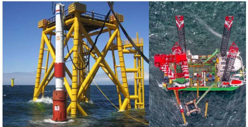
Pile Driving of a Jacket Pile
