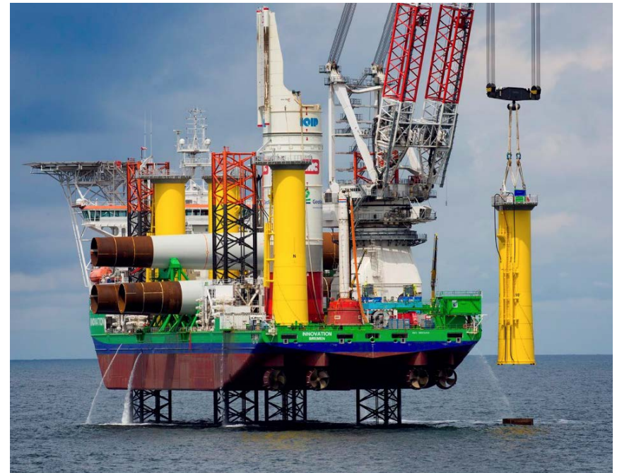
Transition Piece Installation from a Jack-Up Vessel
