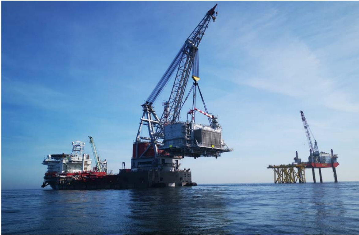
Lifting of Offshore Substation Topside Using Vessel Crane
