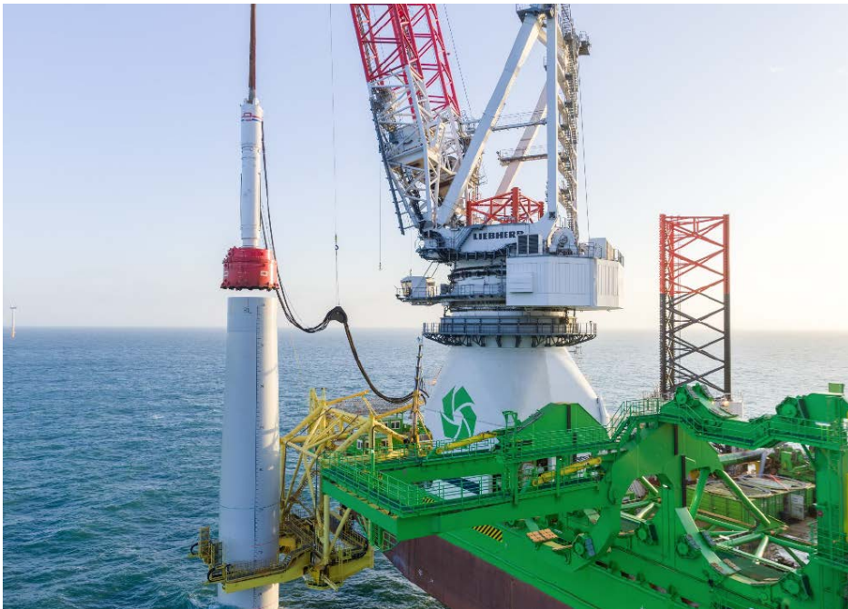
Pile Driving of a Monopile
