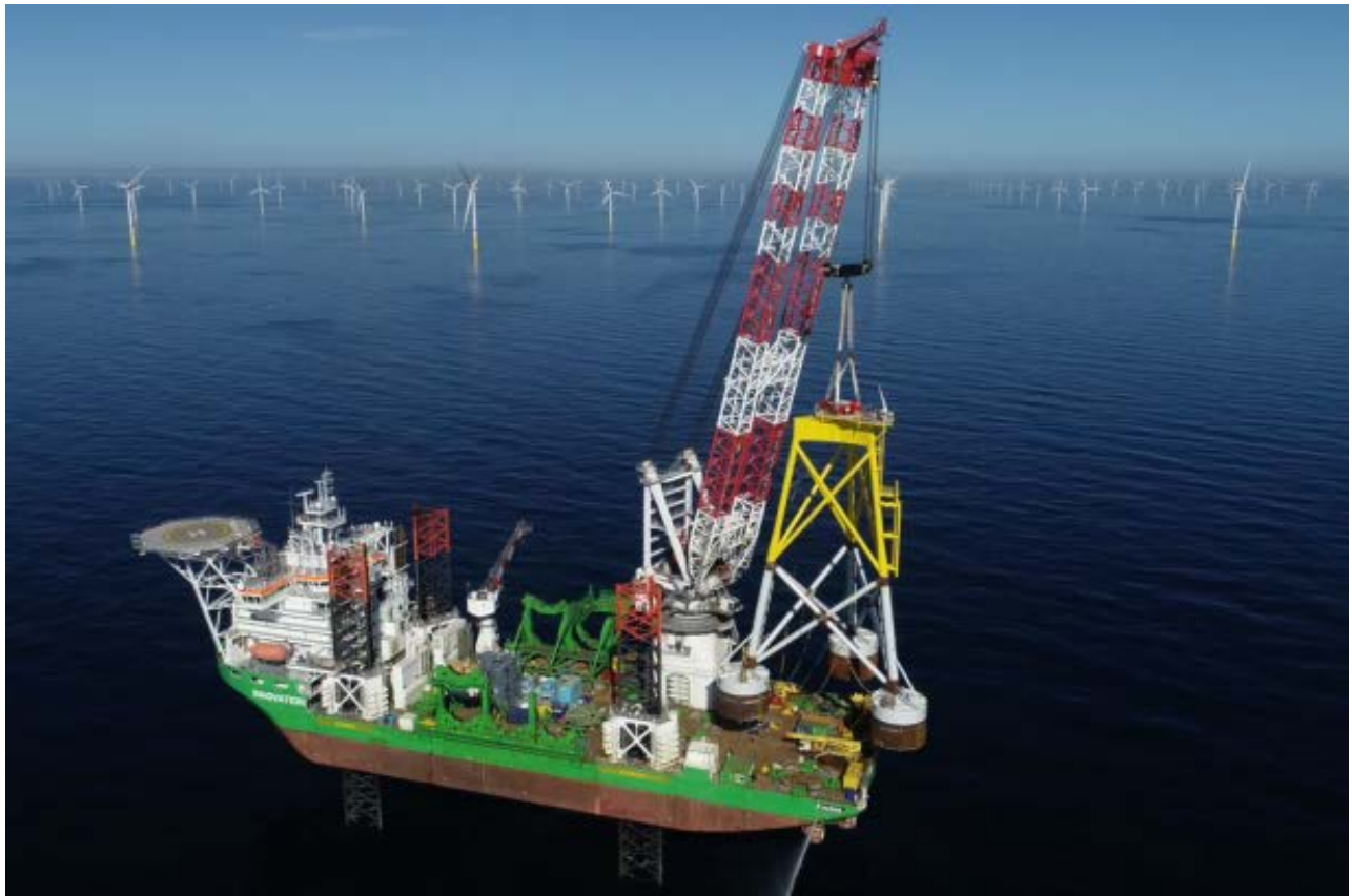
Lowering of Suction Bucket Foundation using Jack-Up Vessel Crane
