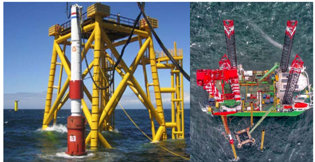
Pile Driving of a Jacket Pile
