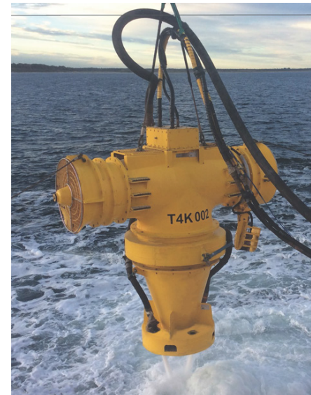
Controlled Flow Excavation
