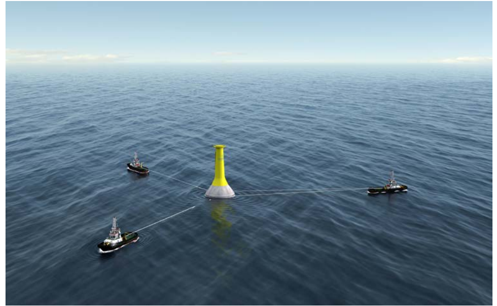
Gravity Foundation Transport via Tugboats
