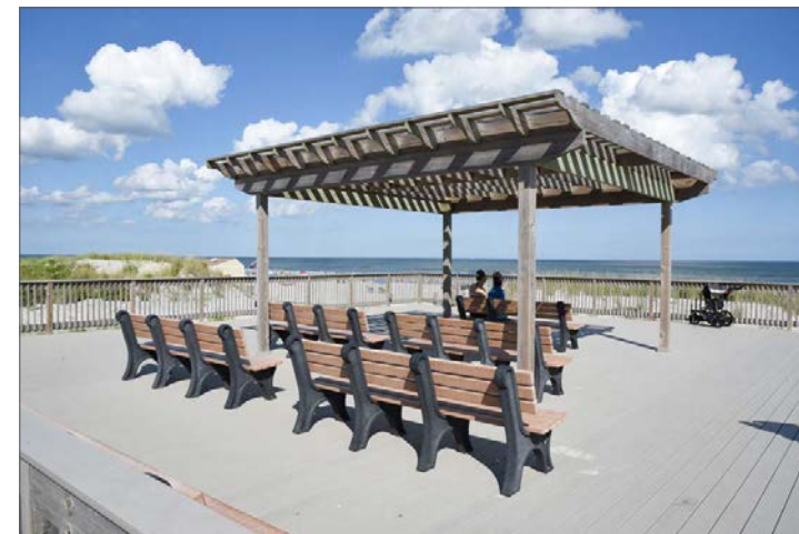
2. View looking east toward gazebo on 95th Street beach access dune viewing platform.
