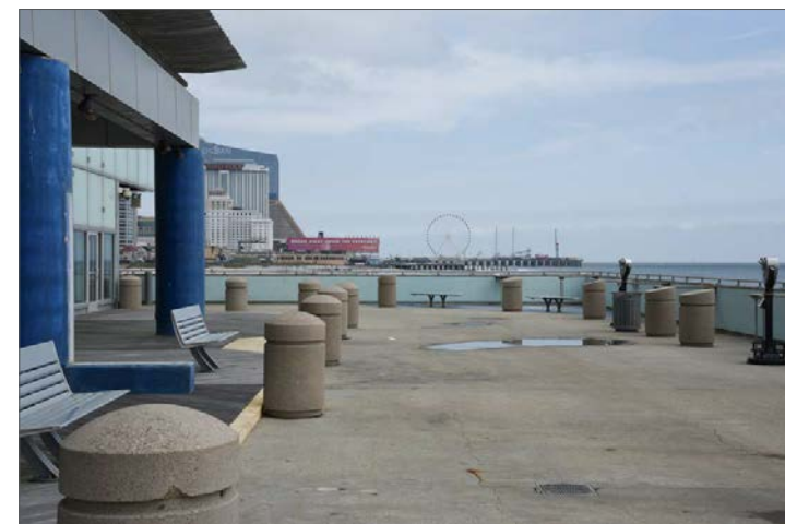
4. View looking northeast from end of playground pier toward Central Pier and Steel Pier.
