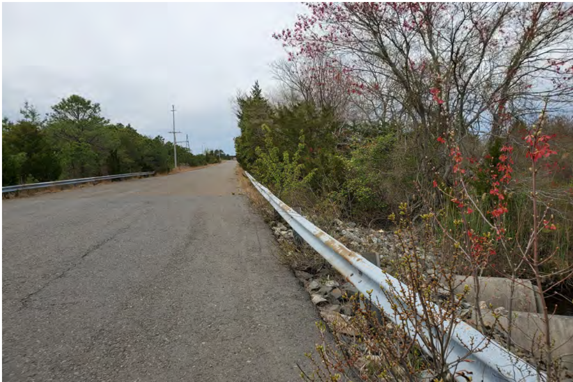
Photo 10: Viewing west along the access road to the Oyster Creek proposed onshore substation.
