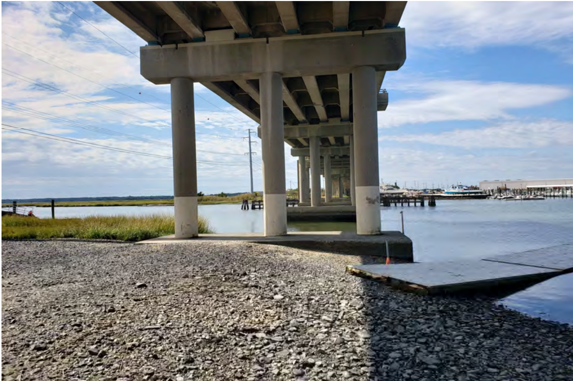
Photo 9: Viewing northwest at the proposed HDD crossing area of Crook Horn Creek, marina in background, public fishing access in foreground right.
