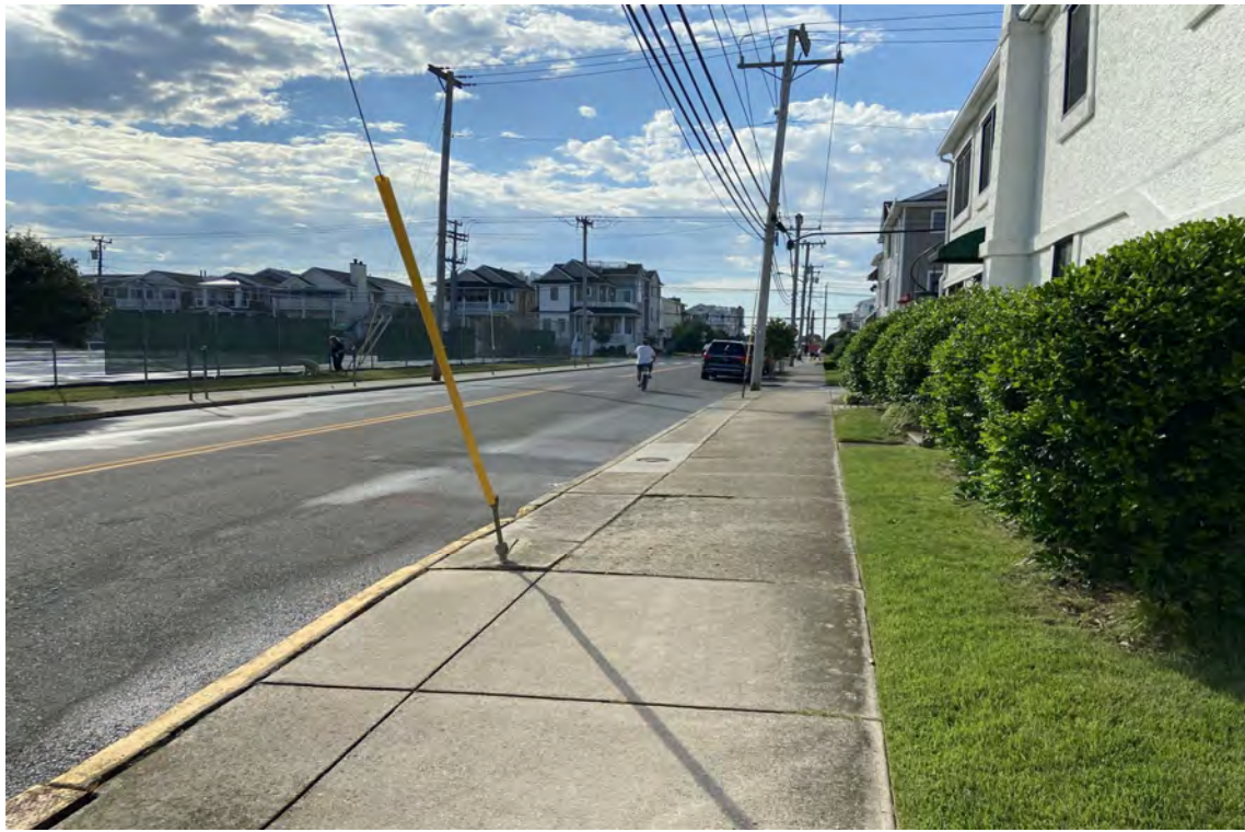
Photo 3: Viewing southeast along 35th Street at the proposed export cable route alignment in Ocean City
