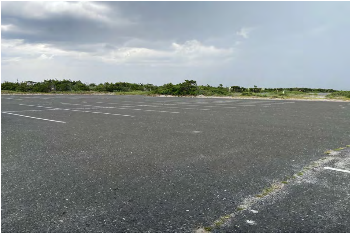
Photo 13: Viewing northwest at the proposed transition joint bay area at HDD landfall at Island Beach State Park
