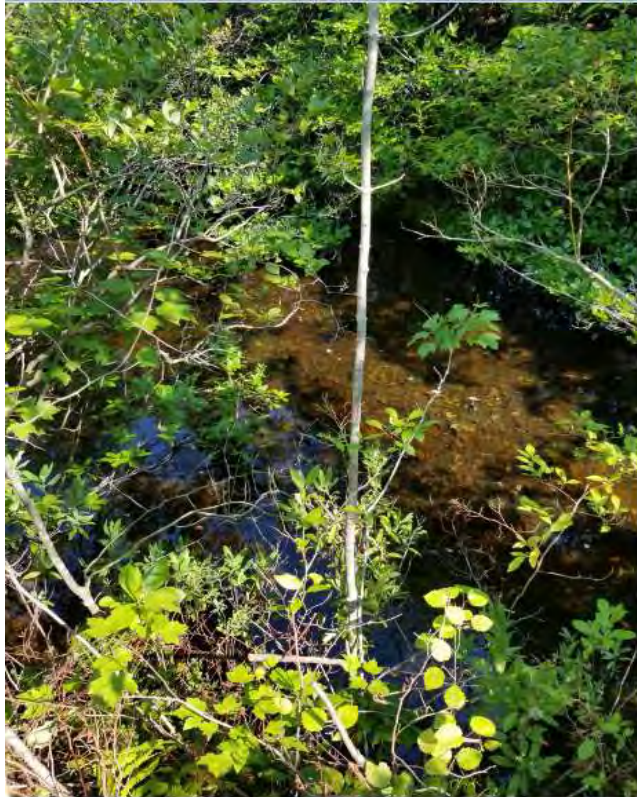
Photo 7: Overgrown/shaded ditch north of main access path east of Route 9.
