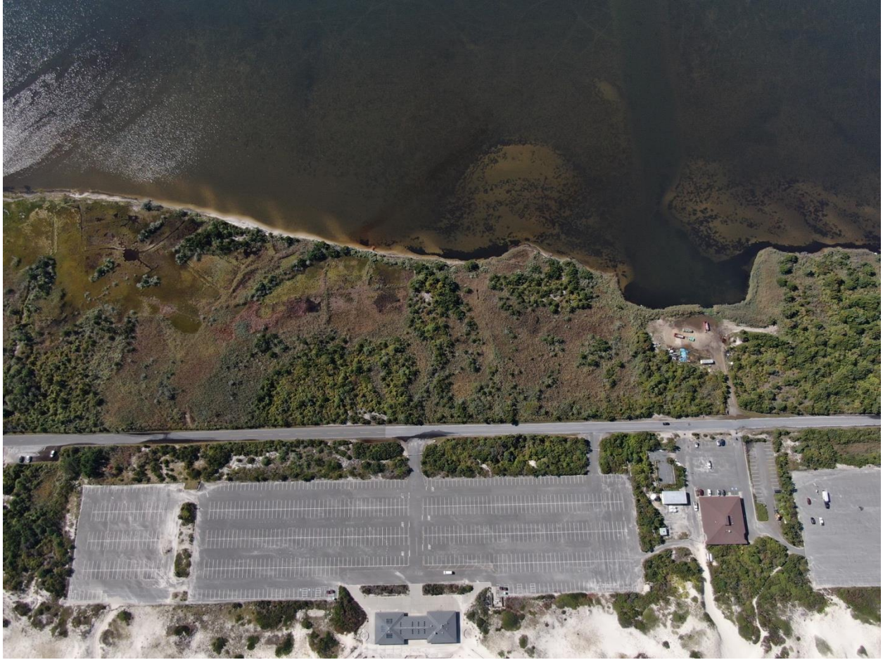
Site photo 3: HDD onshore activities in parking lot behind beach and dune at Island Beach State Park
