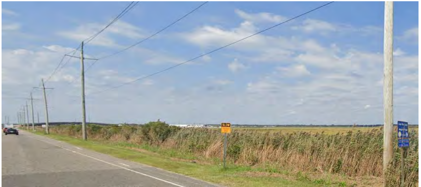
Photo 4: Viewing north along Roosevelt Blvd at proposed export cable route alignment within Ocean City, delineated coastal wetlands adjacent to road.
