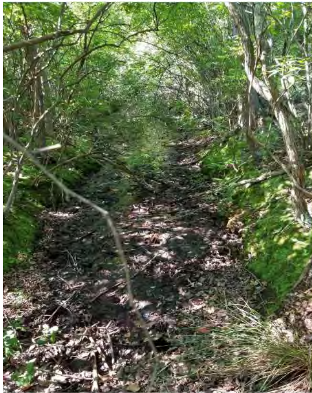
Photo 5: Overgrown/shaded ditch south of main access path east of Route 9.
