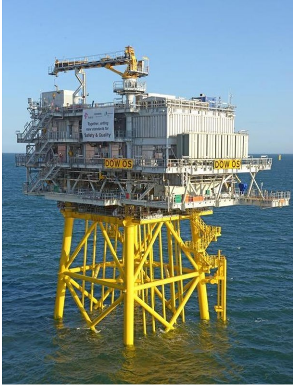
Figure 3-5 Equinor-Operated Dudgeon Offshore Wind Farm: an Offshore Substation Platform on a Suction Bucket Jacket Foundation (Equinor 2021)
