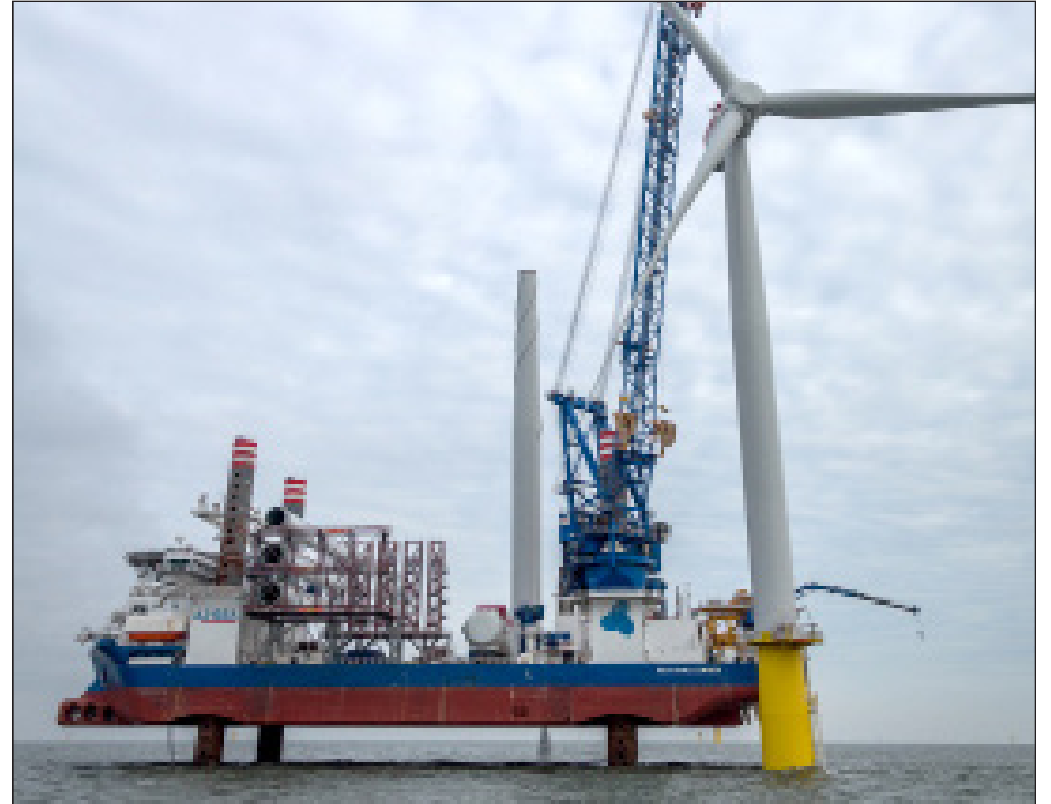
Wind Turbine Installation
