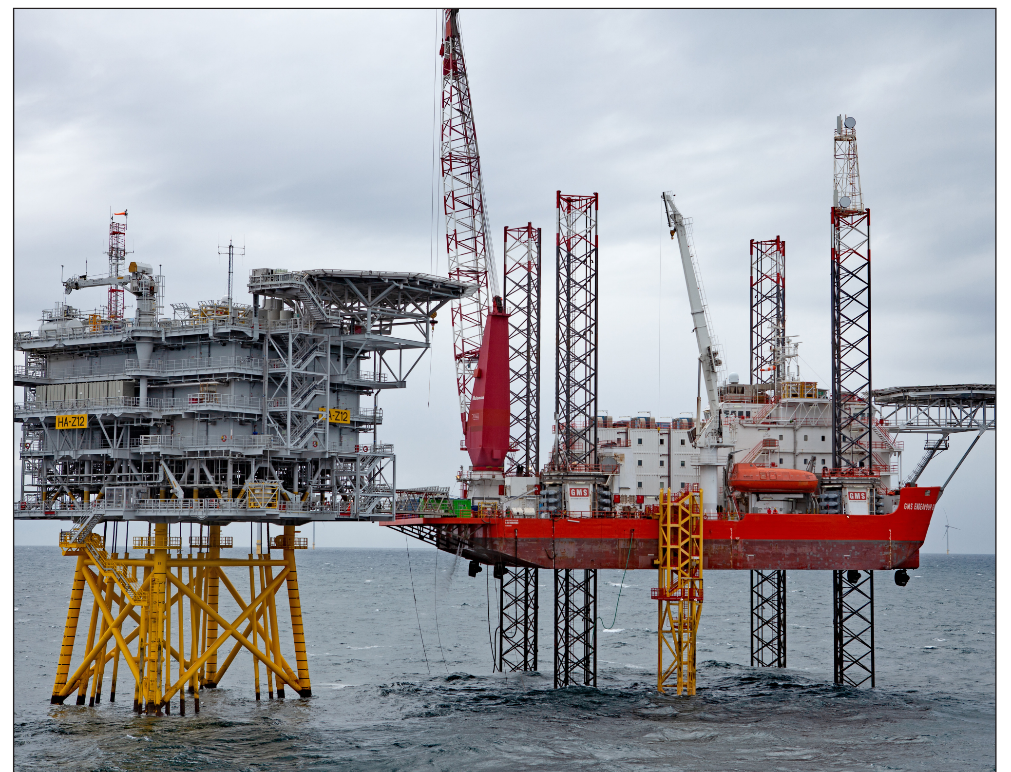
Installation of Offshore Substation
