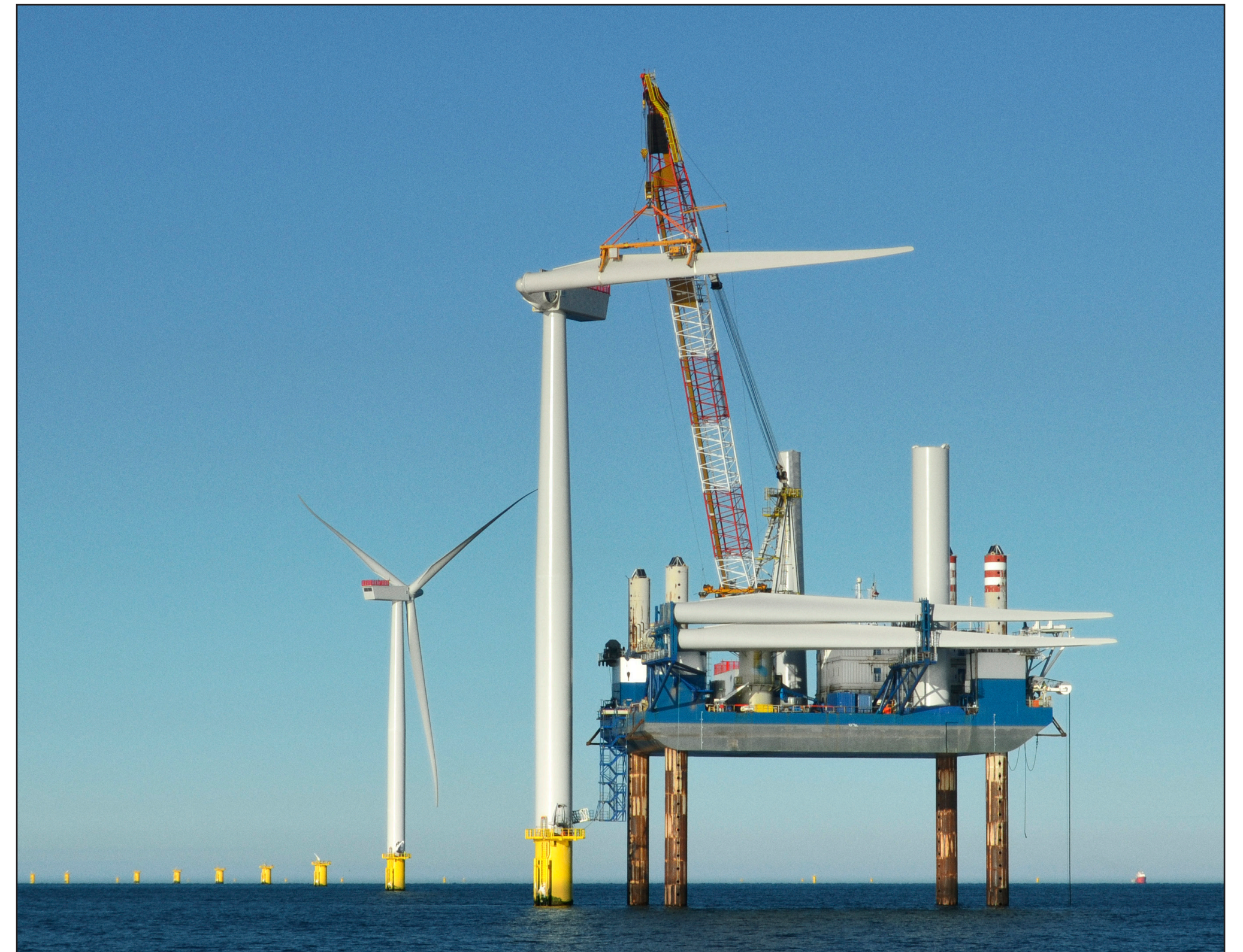
Wind Turbine Installation
