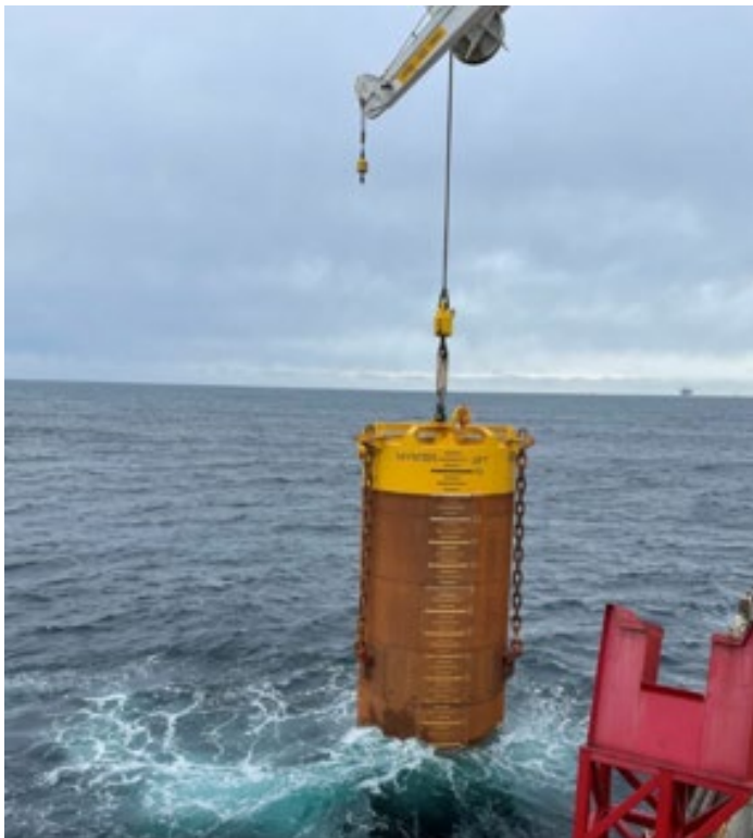
Figure 2-2 Representative Photograph of a Suction Bucket
