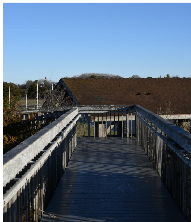
#3 Viewing North, 03/26/2023 8:00 AM
