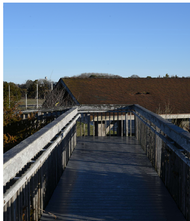
#3 Viewing North, 03/26/2023 8:00 AM
