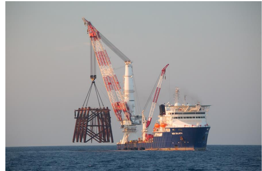
Example of an upper jacket removal Photo credit: BSEE
