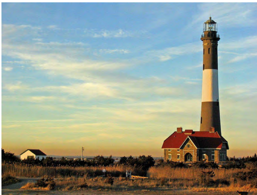
Figure 3-9 Fire Island Lighthouse and Historic District, view to northwest (Source: Wikipedia)
