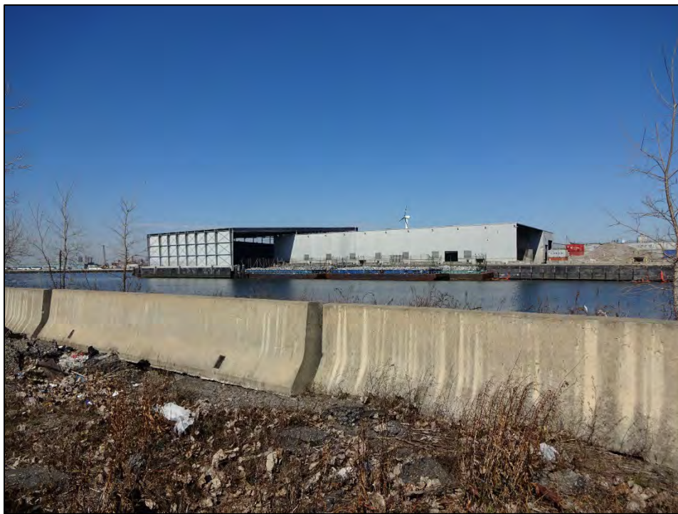
Looking north from 35th Street "Pier" at SBMT toward contemporary recycling facility at 29th Street "Pier." 35th Street "Pier" will be repaved, a wharf installed into the "interpier" basin, and the basin will be dredged, as will the area to the west of the 35th Street "Pier."
