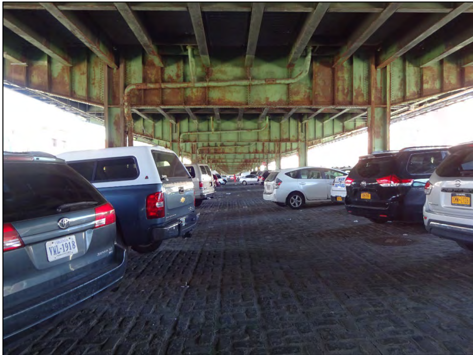
View beneath Gowanus Expressway above Third Avenue.
