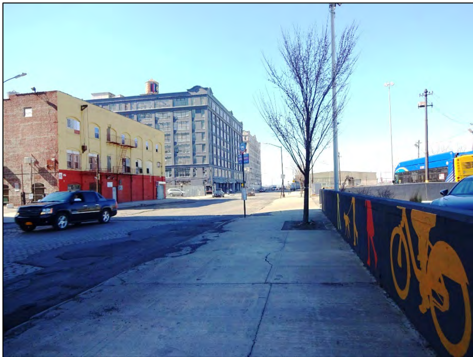
Looking northwest toward Gowanus Bay and SBMT 39 th Street, east of First Avenue. Buildings on left side of photograph are contributing resources within Bush Terminal Historic District.
