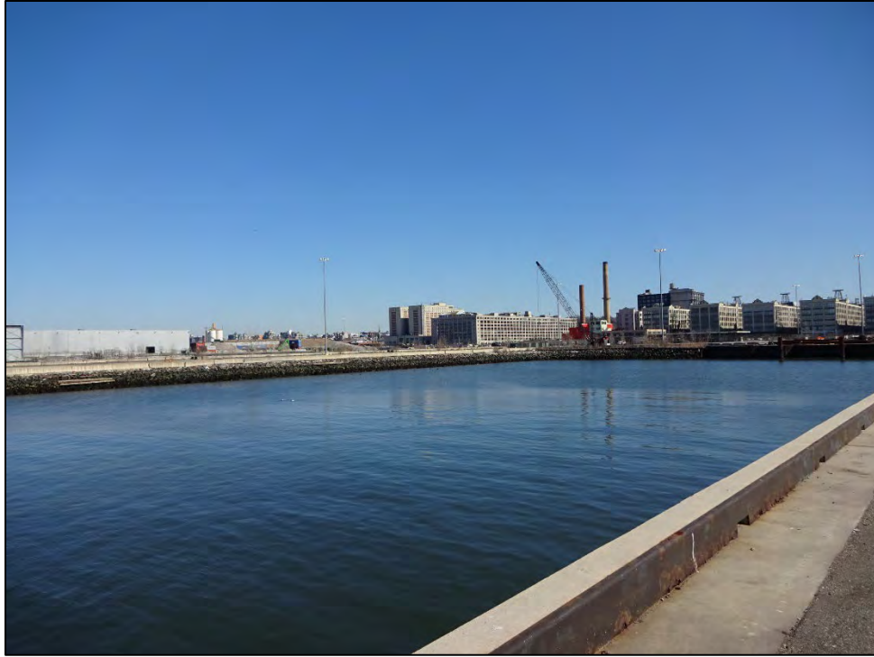
Looking east from 39th Street "Pier" at SBMT toward National Register-listed Navy Storehouse No. 2 (shorter building). "Interpier" basin will be dredged and new paving and structures will be installed.
