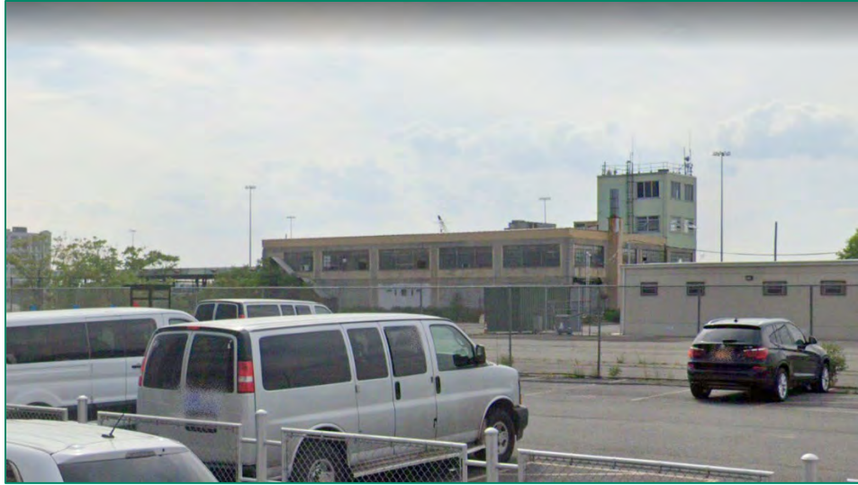
Looking west toward Tower Building at SBMT; building will be removed. Pavement will be removed and new paving and structures installed.
