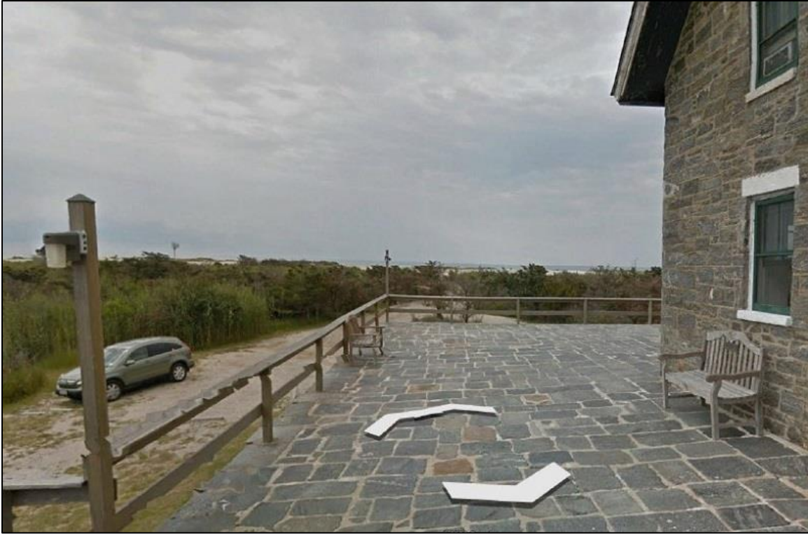
Figure A-7 Fire Island Light Station Historic District in Islip, New York
