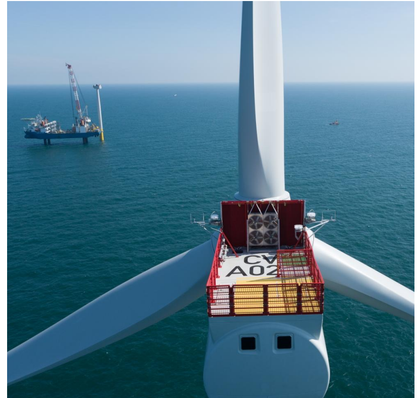
Coastal Virginia Offshore Wind Pilot Project under construction
