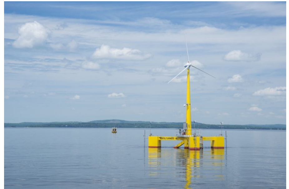
UMaine 1:8 scale floating VoltturnUS foundation
