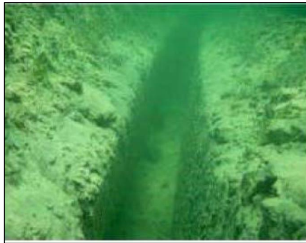
Figure 2.3.2-10. Example of a Cable Trench (Latham et al. 2017).
