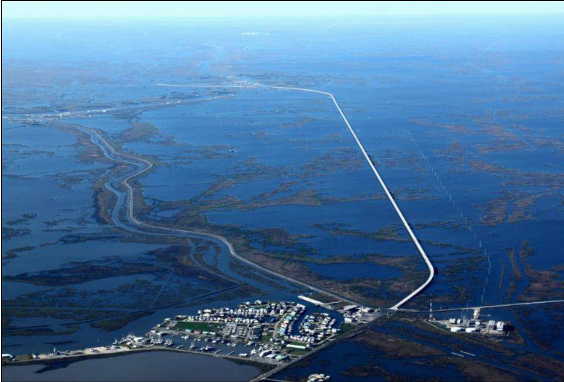
Figure 4.4.1-7. LA Hwy 1 Connecting Port Fourchon and Leeville, Louisiana (Photo Credit: (LA 1 Coalition 2018)). The new elevated highway is bright white and the old LA 1 is the curving road to its left. Port Fourchon is visible at the bottom of the photo.
