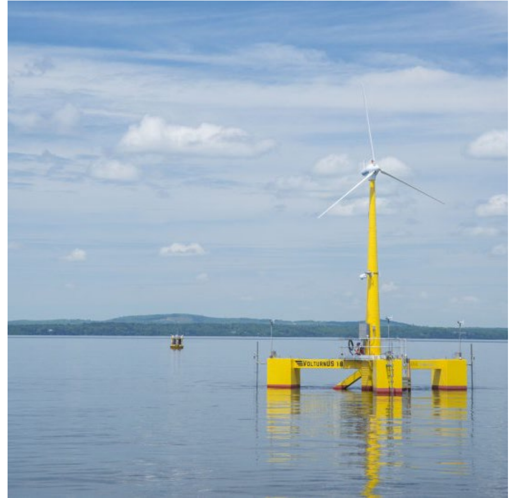
UMaine 1:8 scale floating VoltturnUS foundation
