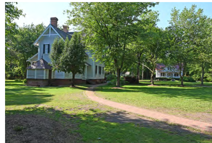
1. The original Keeper's Quarters at the base of the lighthouse is now the Currituck Beach Lighthouse Museum.
