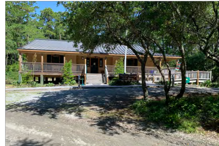
1. Park Visitor Center, 1.1 km (0.7 mi) west of the ocean, features interpretive displays, supplies, and toilet facilities.
