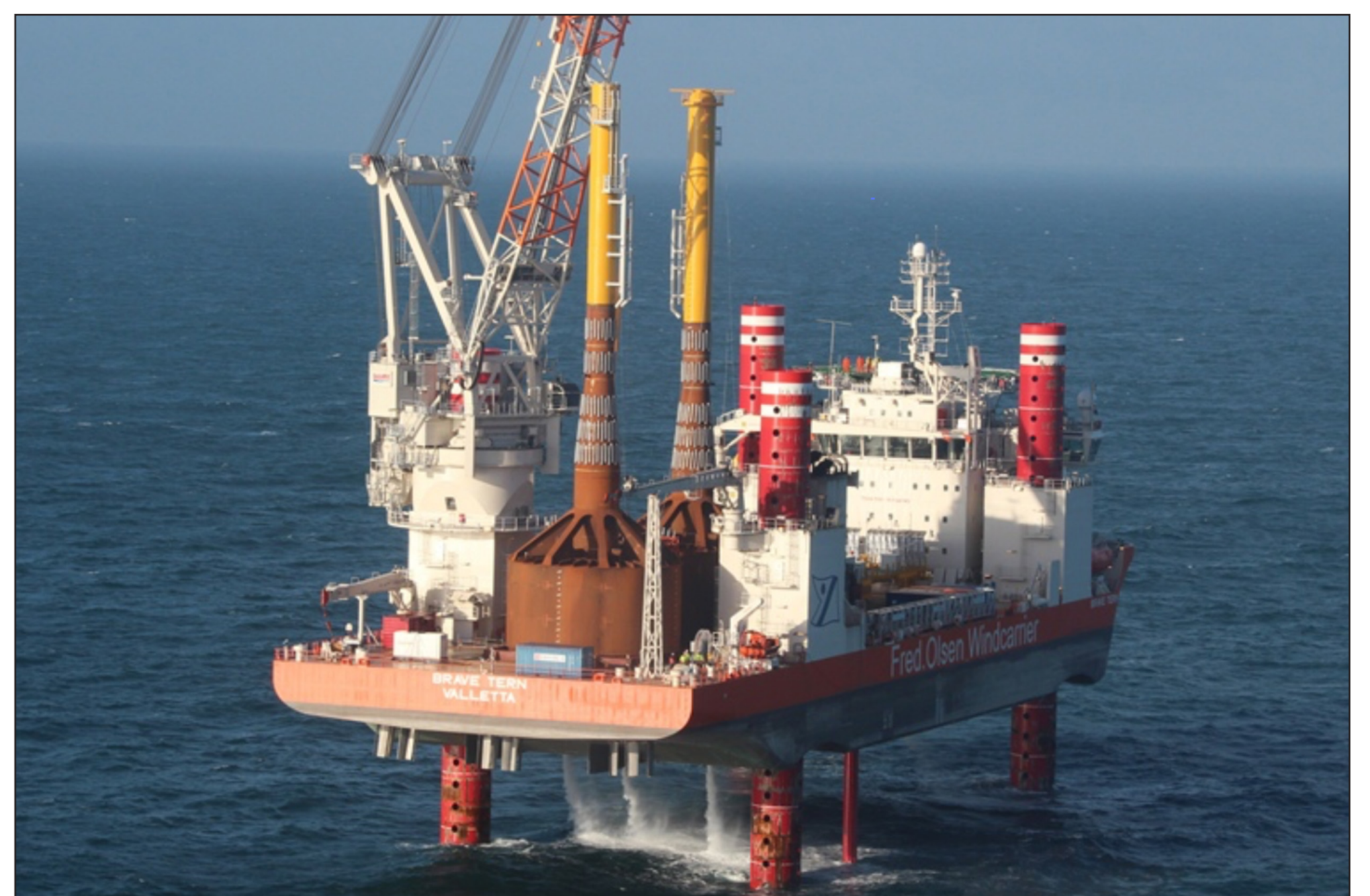
Offshore transportation of monobucket on jack-up vessel
