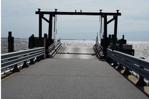
Ferry landing, Currituck NC on the western shore of Currituck Sound.
