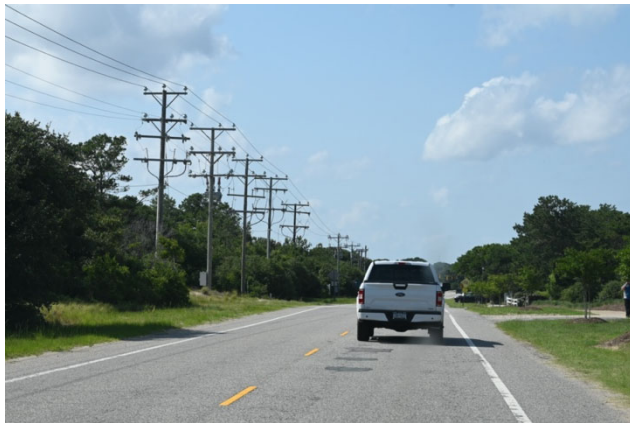
Wire utilities paralleling Route 12 in Corolla.
