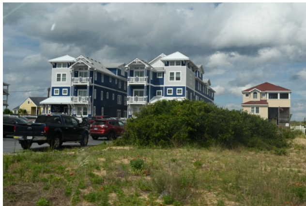
Many small cottages have been removed to make way for multi-story multi-family vacation homes.
