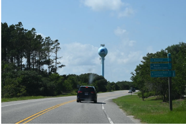
Water tower with co-located communications equipment, Currituck.
