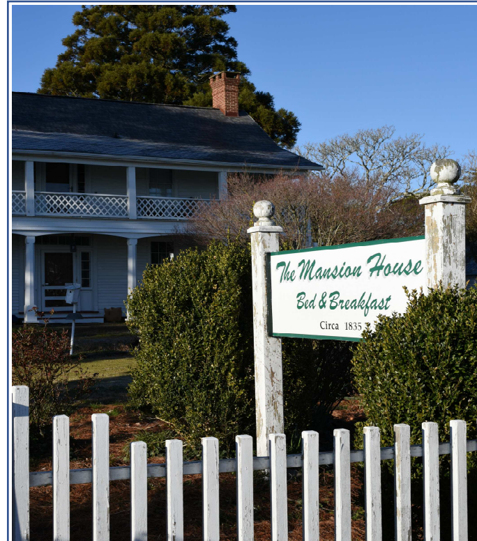
#1 Context Photo, 03/21/2023 8:30 AM A view of the Mansion House bed and breakfast, taken from the public parking lot.
