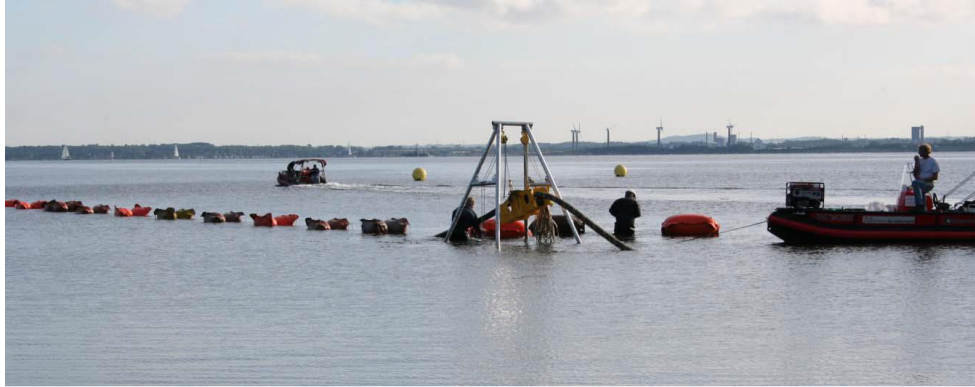
Figure 3-12. Example of Shallow Water Cable Installation
