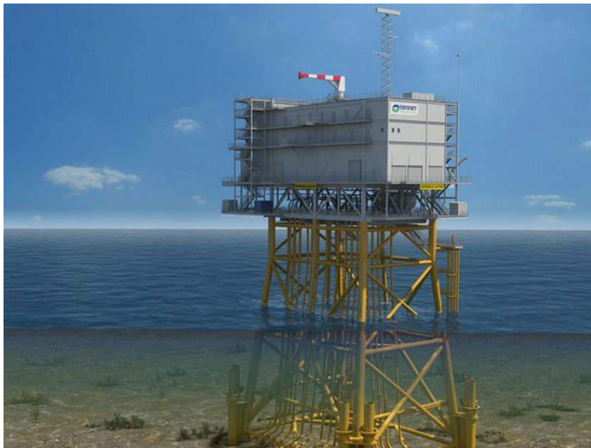
Figure 3-3. Example High-Capacity OSS with Jacket Foundation and Skirt Piles
