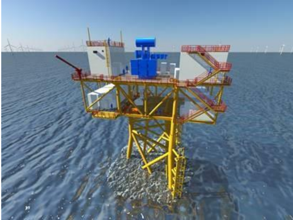
Figure 2-7. OSS on Jacket Foundation Source: HSM Offshore
