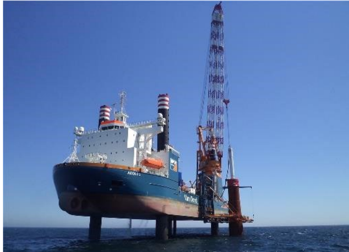
Figure 3-2. Monopile Installation Source: Globalenergyworld.com
