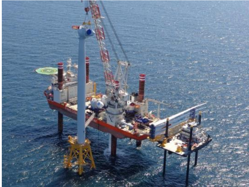
Figure 3-17. Offshore WTG Installation Vessel Source: blockisland.com
