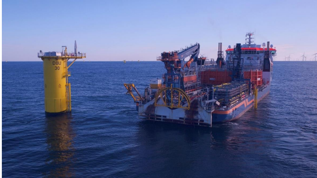
Figure 3-14. Dynamically Positioned Cable Installation Vessel Source: Deutsche Bucht and Van Oord
