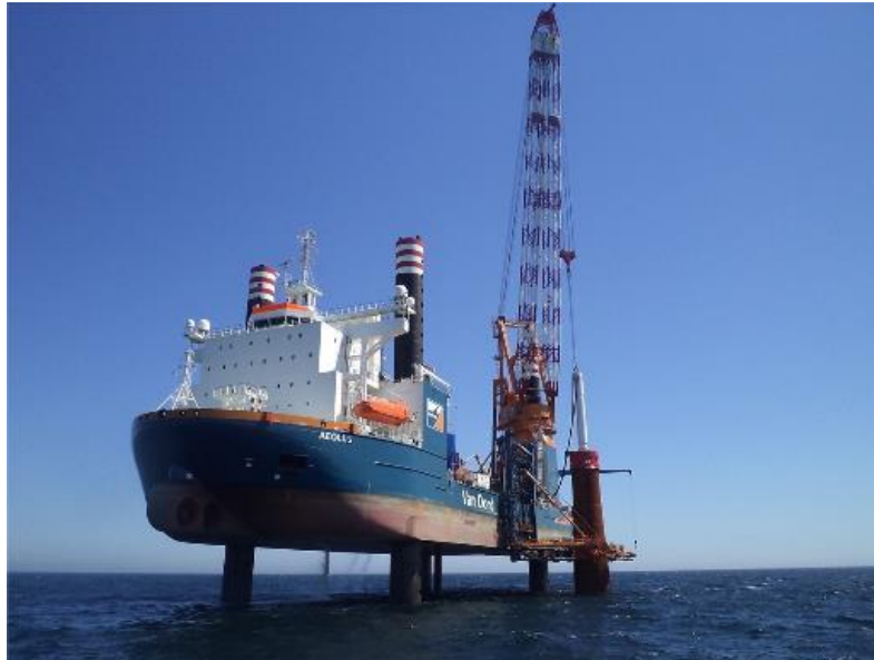
Figure 3-2. Monopile Installation Source: Globalenergyworld.com
