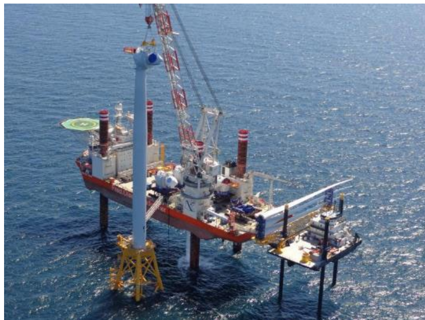
Figure 3-17. Offshore WTG Installation Vessel Source: blockisland.com
