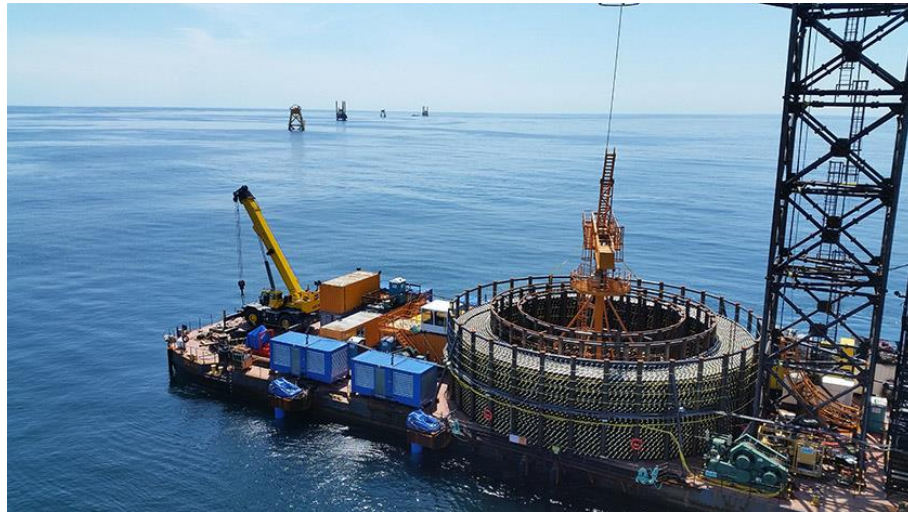
Figure 3-11. Block Island Cable Installation Source: www.oceannews.com
