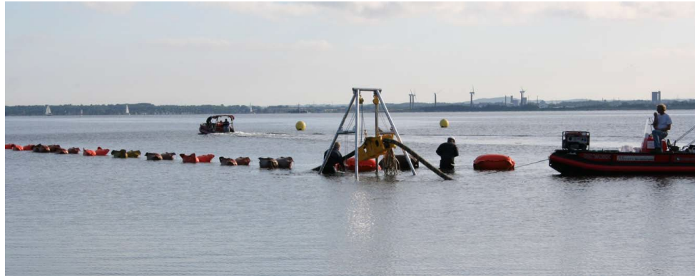
Figure 3-12. Example of Shallow Water Cable Installation
