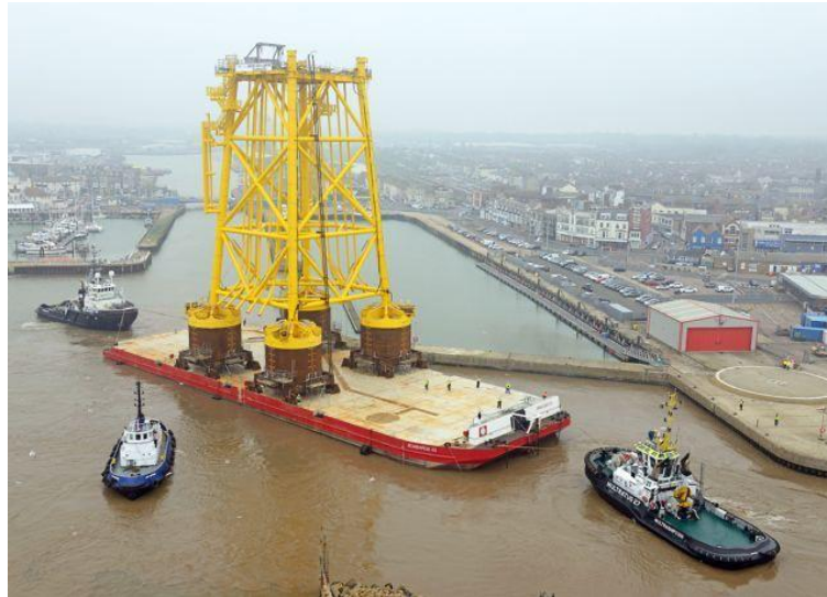
Figure 3-4. Jacket on Suction Bucket Transport Source: www.chpv.co.uk
