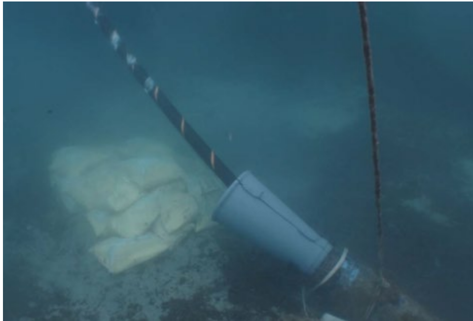
Figure 3-9. Underwater View of Near Shore Cable Pull into HDD Duct Source: Nexans.com
