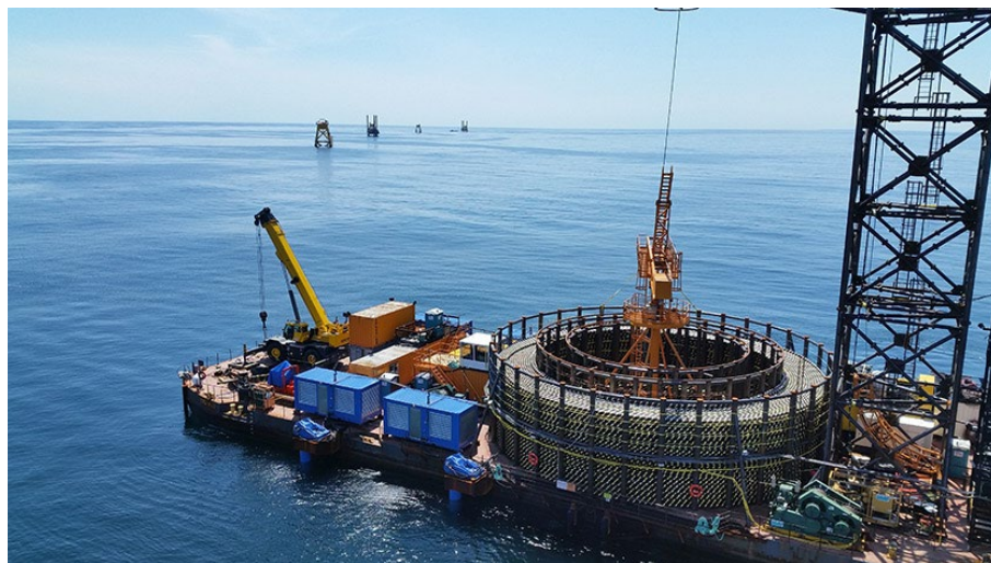
Figure 3-11. Block Island Cable Installation Source: www.oceannews.com
