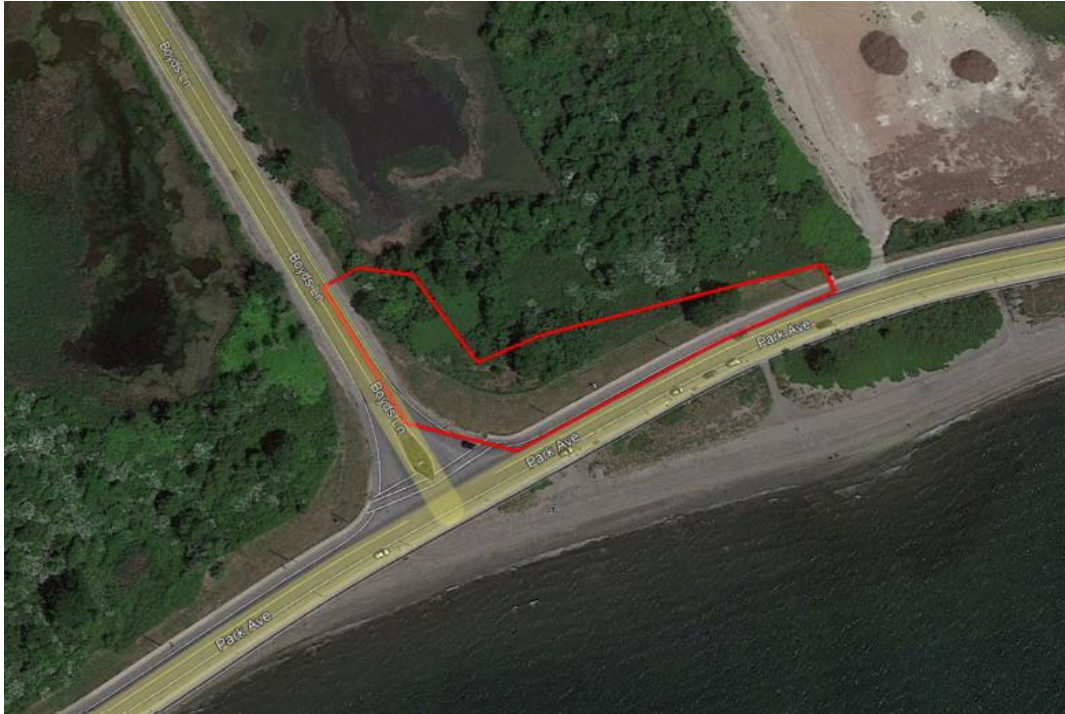
FIGURE 12-9. INTERMEDIATE LANDFALL ENTRY HDD – AQUIDNECK ISLAND
