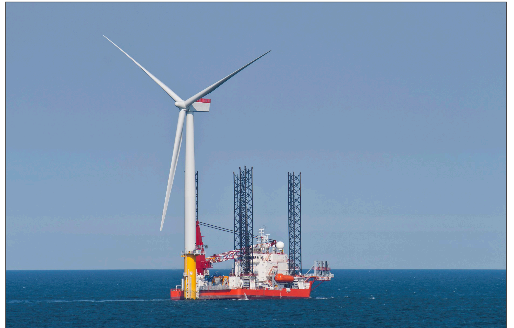
Jack-up Vessel Installing a Wind Turbine Generator (Source: DNV 2021)
